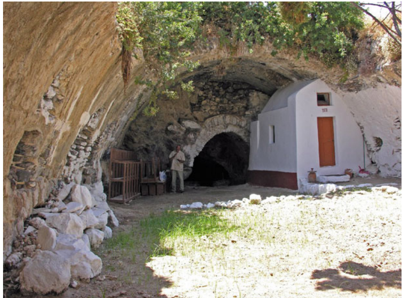
Fig. 12.10 The vault of the Roman thermal bath of the spring Panagia Thermiani east of Pali. Photo community of Nisyros
