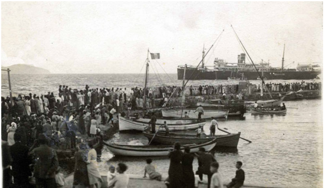
Fig. 12.20 The reinforced pier at Mandraki harbor 1920. Unknown photographer
