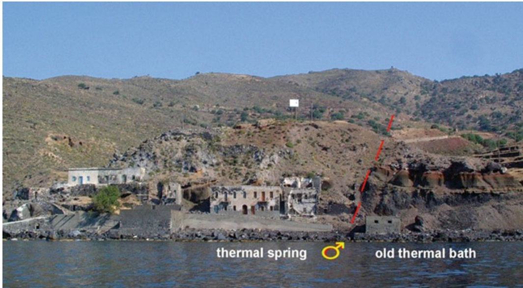
Fig. 5.34 Avlaki's old thermal bath, destroyed by southern winter storms and earthquakes. The thermal spring marks the steep westward dipping N-S fault. Photo V. Dietrich
