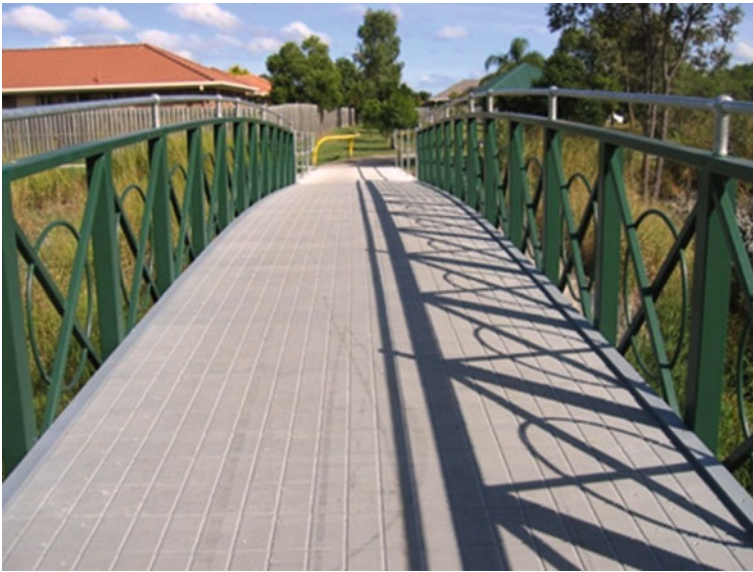
Photo 6.8 Plastic packaging can be reprocessed into different products such as plastic ‘lumber’: example of ‘open loop’ recycling (Photo: Replas)
