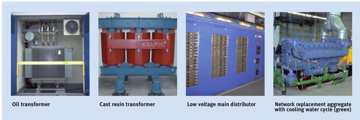
Fig. 3-54 Aggregates for power supply
