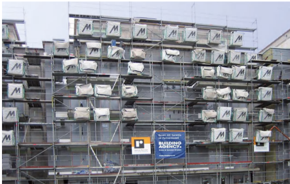
Fig. 4-47 Assembly bags for insulation work on the scaffolding
