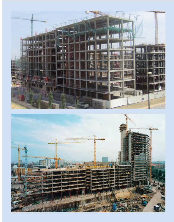
Abb. 3-11 Reinforced steel skeleton construction
