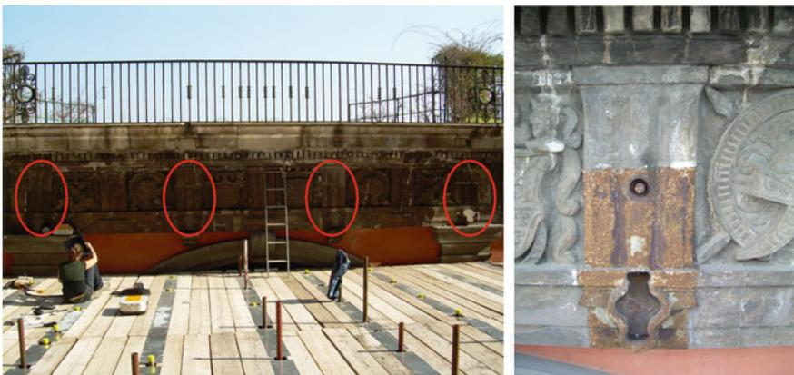
**Fig. 4.12** Location of the 4-iron pins on B-Wall to the left and detail of the hinge on the right
