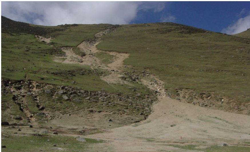
Fig. 5.7 Right-side slope debris flow at DK1927+720
