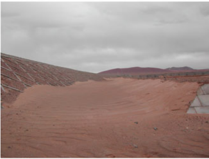
e. Depositing sand on right subgrade of Xiushui River Bridge
