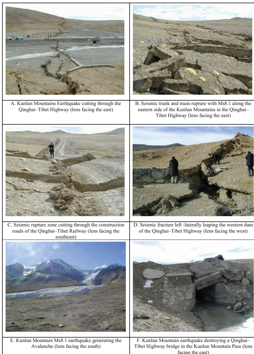
Fig. 4.16 Damage of Kunlun Mountain Ms8.1 earthquake
