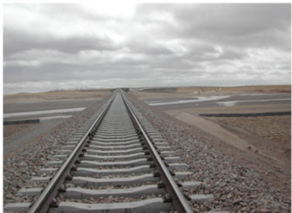
f. Depositing sand on toe of subgrade of Tongtian River Bridge
