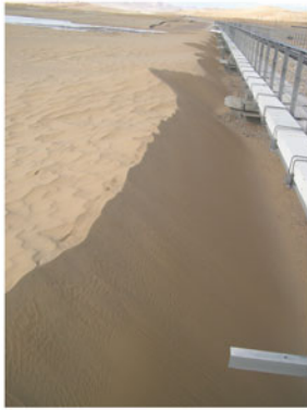
a. Depositing sand under Basuqu Bridge
