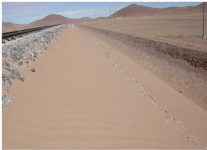
c. Depositing on left between 1476+160 to DK1477+400
