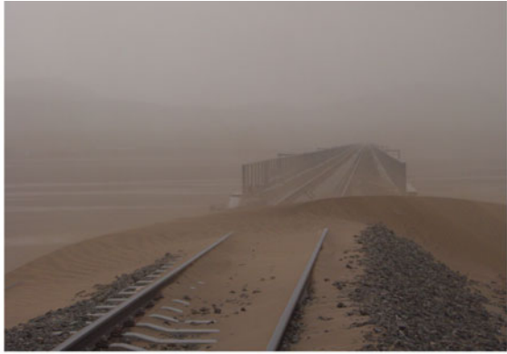
b. Depositing sand on subgrade of sbtument of Tuotuo Bridge
