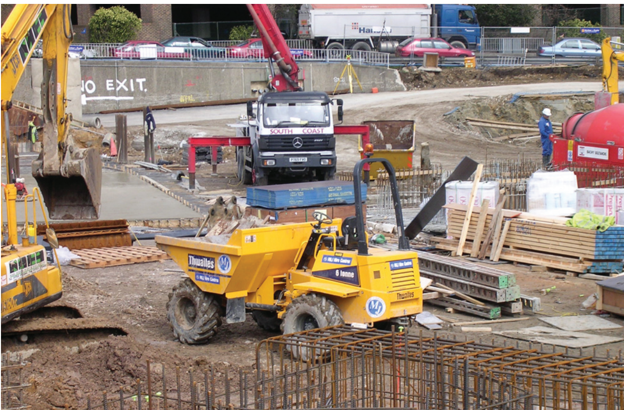
Figure 11.10 Dumper truck with roll-over protection.
