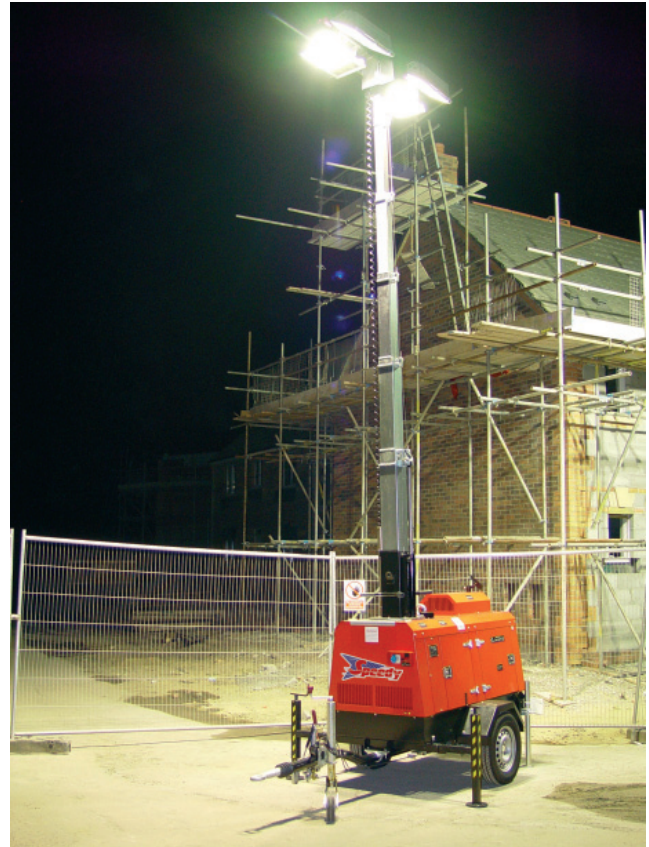
Figure 17.6 Well-lit construction site at night.
