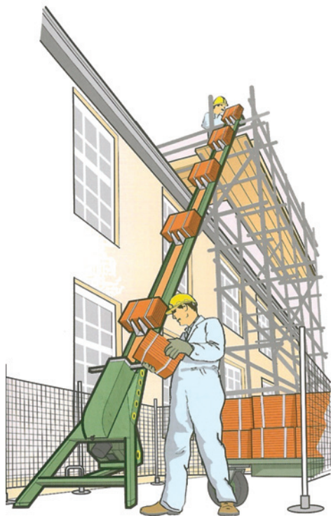
Figure 13.9 A brick elevator.
