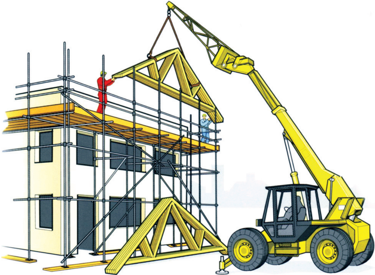
Figure 13.11 Lifting roof trusses.
