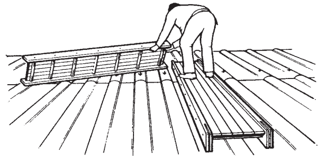
Figure 8.4 Proper precautions must always be taken when working on or near fragile roofs.
