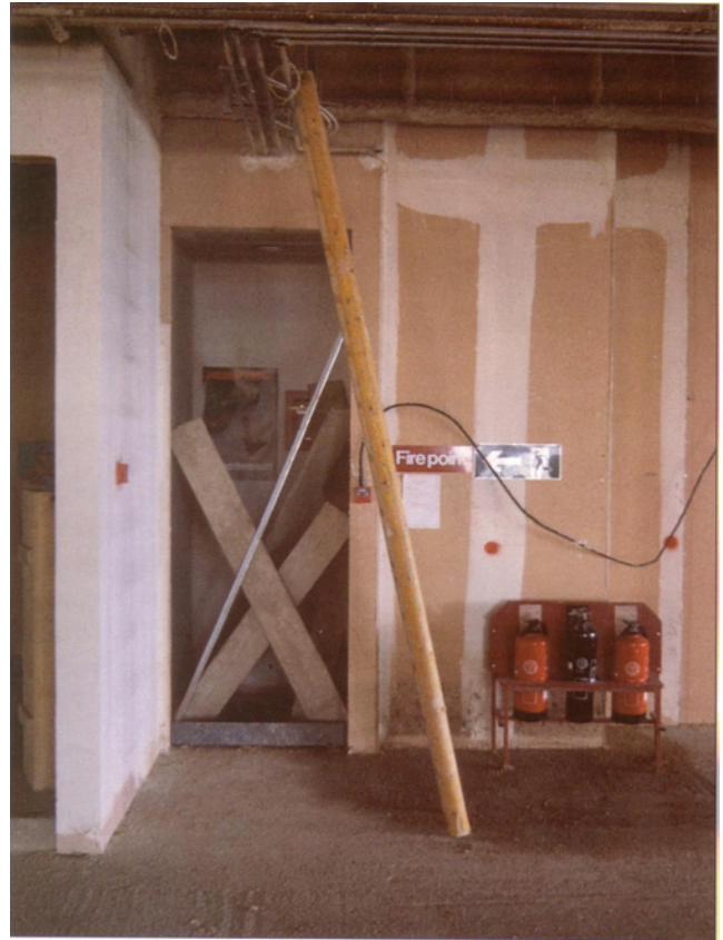
Figure 15.10 This means of escape has been blocked off and will be useless in the confusion of a fire.
