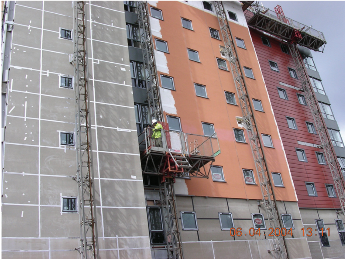
Figure 8.1 Working at height – mast climbing platforms.
