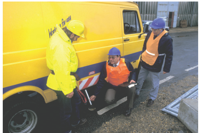
Figure 3.6 Contractors at work.
