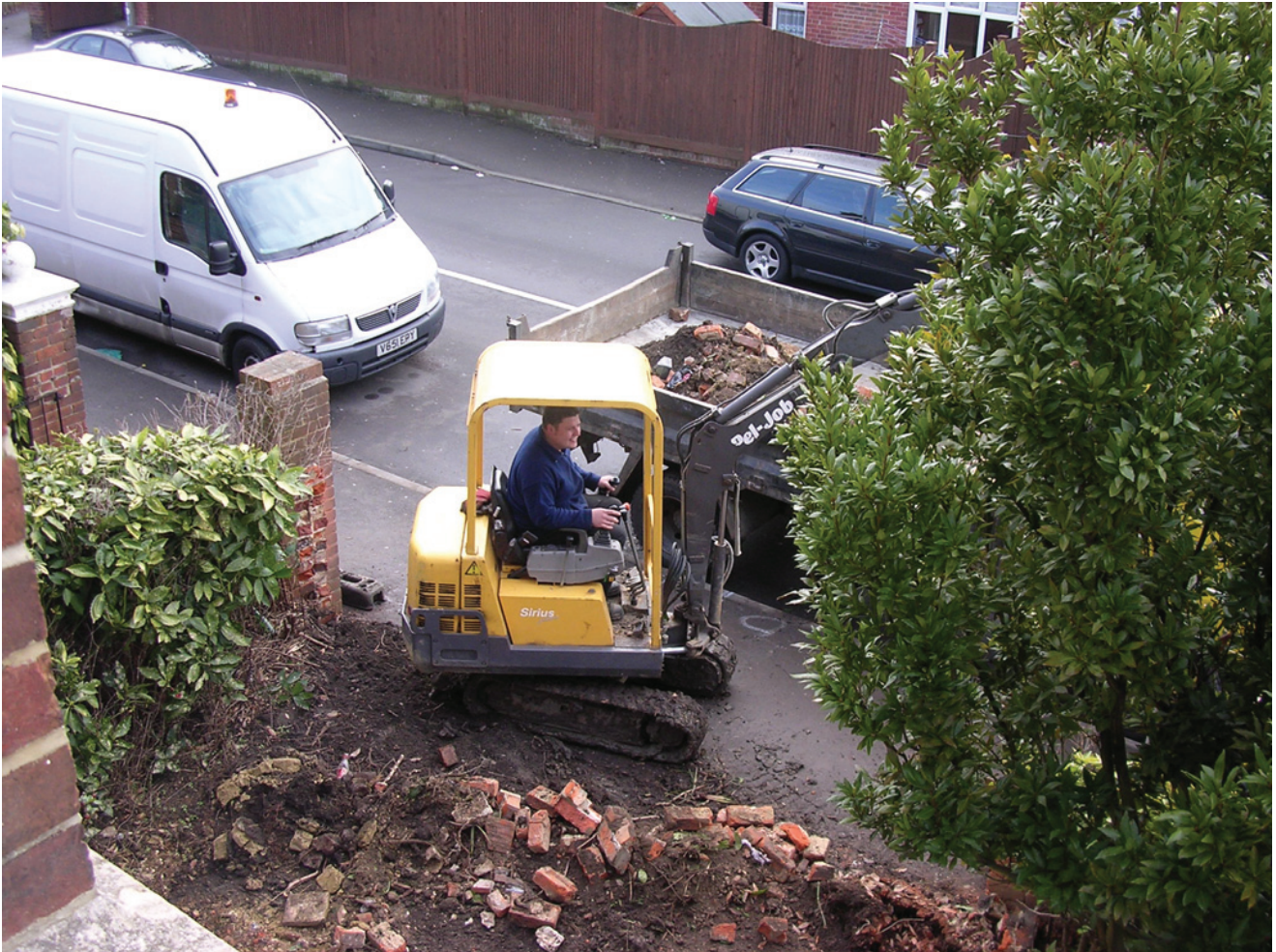
Figure 11.12a Small builders often use the road without taking precautions, and have a wide variety of road vehicles.
