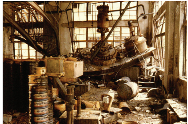
Figure 18.1 A dangerous occurrence – fire.
