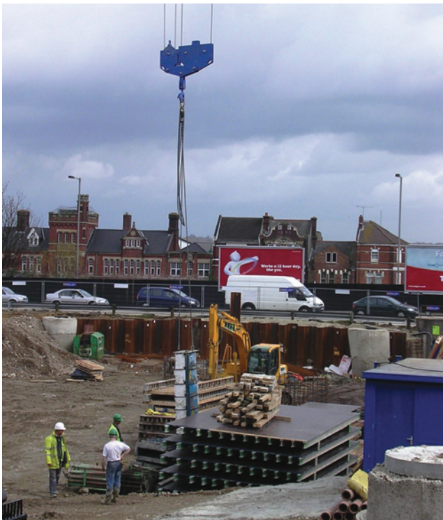
Figure 13.1 Handling on a construction site.
