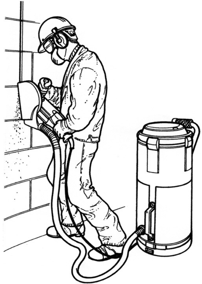
Figure 6.2 Good dust control for a chasing operation. A dust mask is still required for complete protection.
