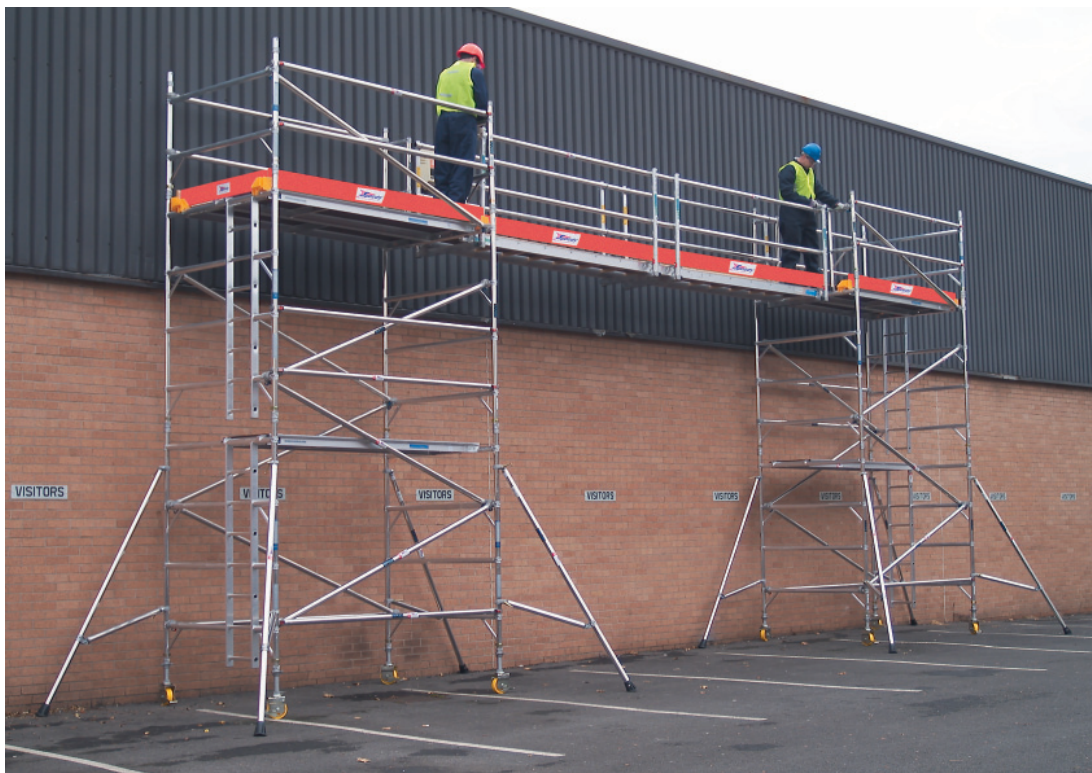
Figure 8.2 Working platform, tower scaffolds and bridging units.
