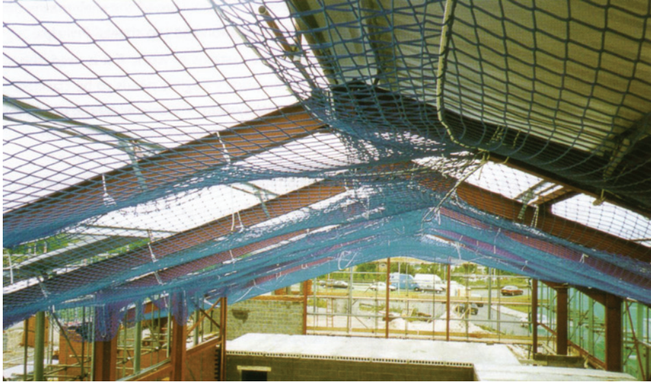
Figure 8.3 Industrial roof work: use of safety nets.
