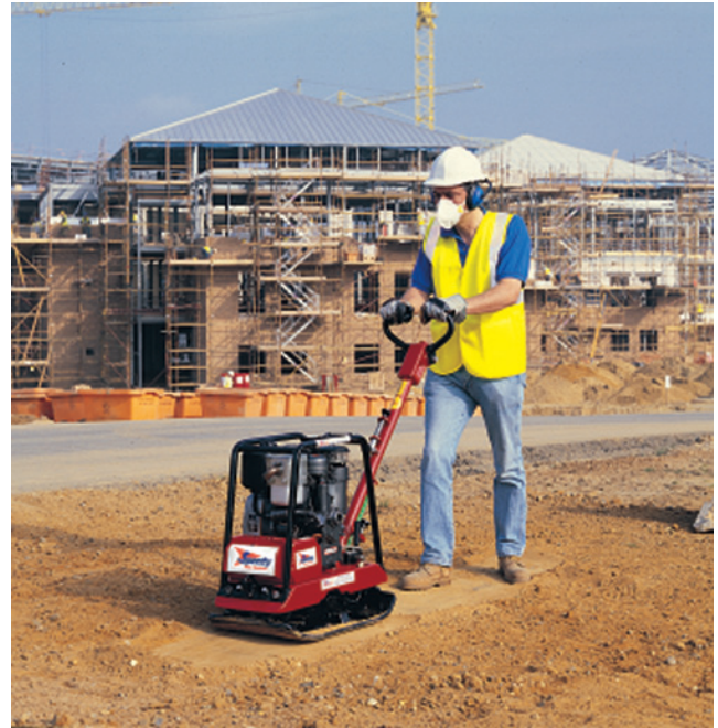
Figure 12.25 Plate compactor.
