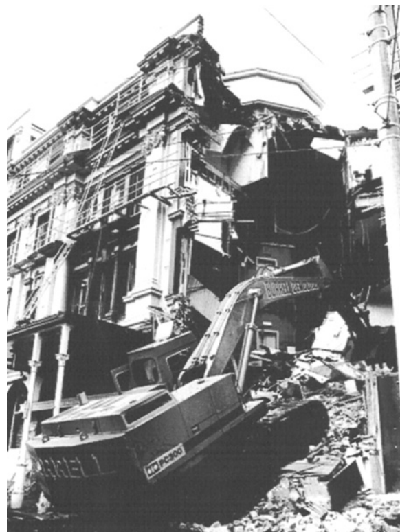
Figure 10.1 Demolition in progress.
