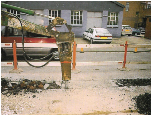
Figure 17.4 Mounted breaker to reduce vibrations.
