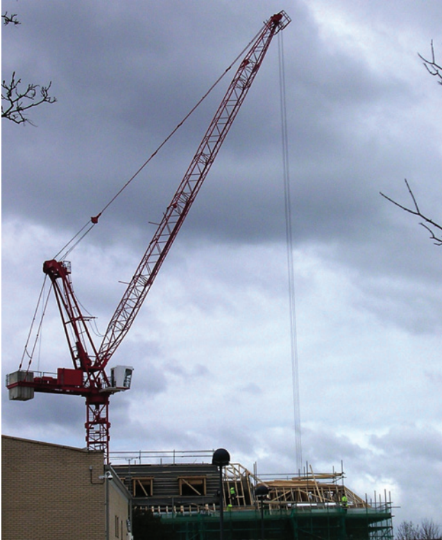
Figure 13.13 Typical jib tower crane.
