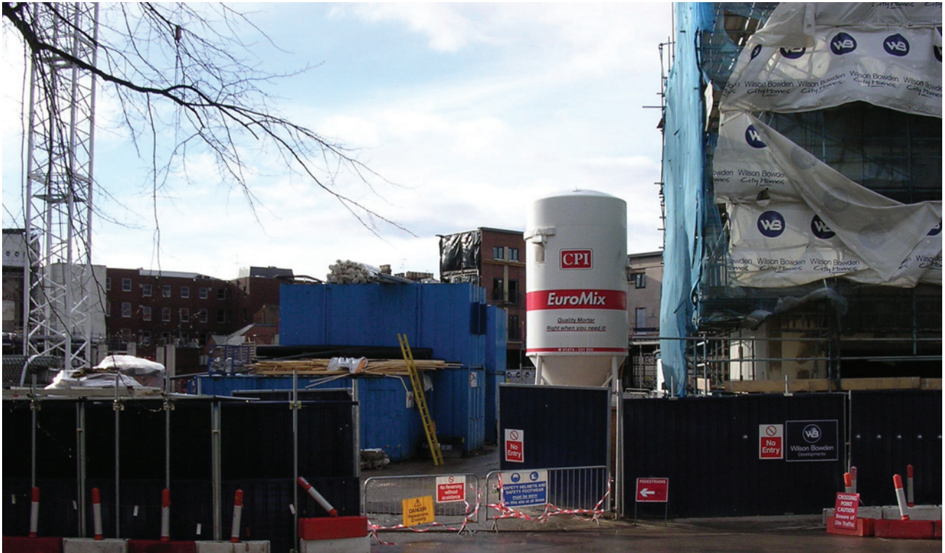
Figure 7.1 Typical construction site.
