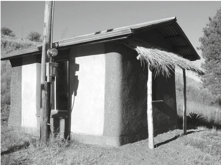
Figure 6.4 The Pumphouse, a demonstration straw-bale shed at the Canelo Project
