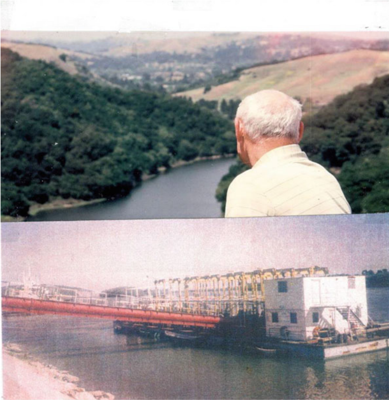
Fig. 41.5 A dam up of a surface to be irrigated (California, USA) and a floating pumping station below the surface to be irrigated (Constanta county, Romania, on the Danube river) (Source: Aurel Lup's personal photo archive)
