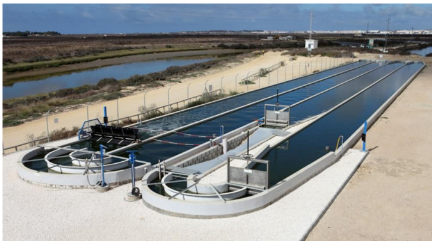
Figure 4.3 Raceway ponds installed in Chiclana de la Frontera (South Spain) with two different configurations: conventional mixing by paddle wheels (left) and innovative patented raceway mixed by propeller with modified bends (right).
