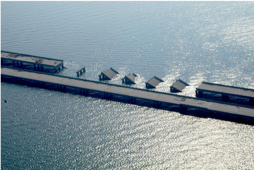
**Figure 21.1.** New Orleans, September 20, 2005. Sections of the eastern span of a causeway slid off their moorings and into the lake due to the winds and waters of Hurricane Katrina. (Photo: Win Henderson, Federal Emergency Management Agency (FEMA).)
