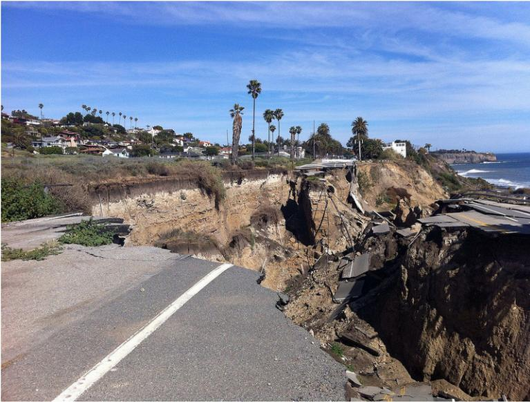
**Figure 20.1.** Landslide near San Pedro, California, on November 21, 2011. Rain exacerbated a slow-moving landslide that left large crevices on a road along the coast. The road broke into pieces that crumbled into gaping holes, while other sections fell into the ocean below. (Photo: USGS: US Geological Survey, [www.gallery.usgs.gov/afv2YLk885/large/san\\_pedro\\_landslide\\_knabe.jpg](http://www.gallery.usgs.gov/afv2YLk885/large/san_pedro_landslide_knabe.jpg).)
