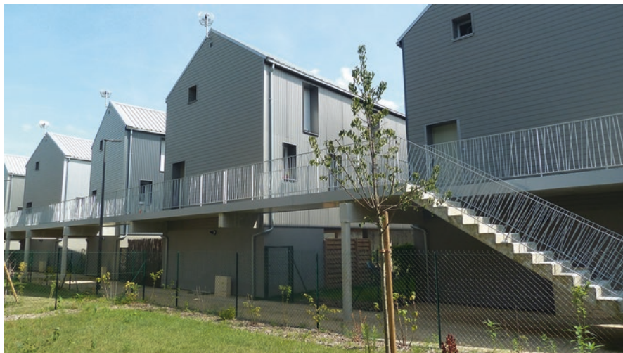
Fig. 11.1 Flood adapted passage way in St Pierre de Corp
