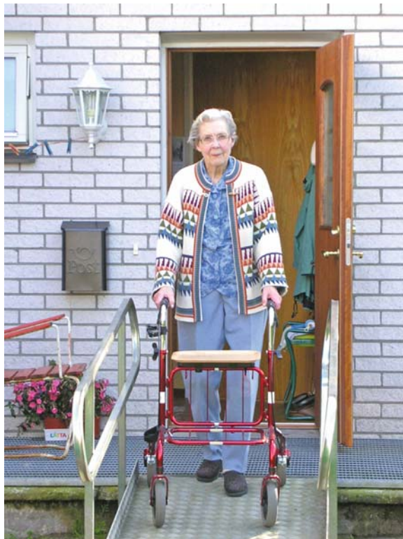
Fig. 5.1 Installation of ramps at entrances is among the most common housing adaptation measures. (Photograph: S. Iwarsson; reproduced with the subject’s approval.).
