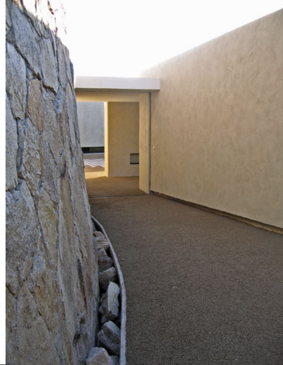
Entry into a compressed gateway to the compound.
