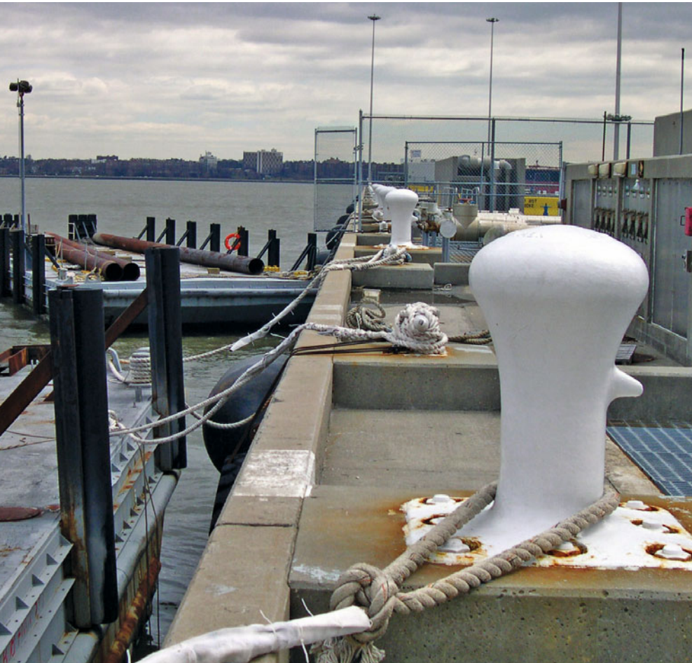
Existing bulkhead, Stapleton, Staten Island.
