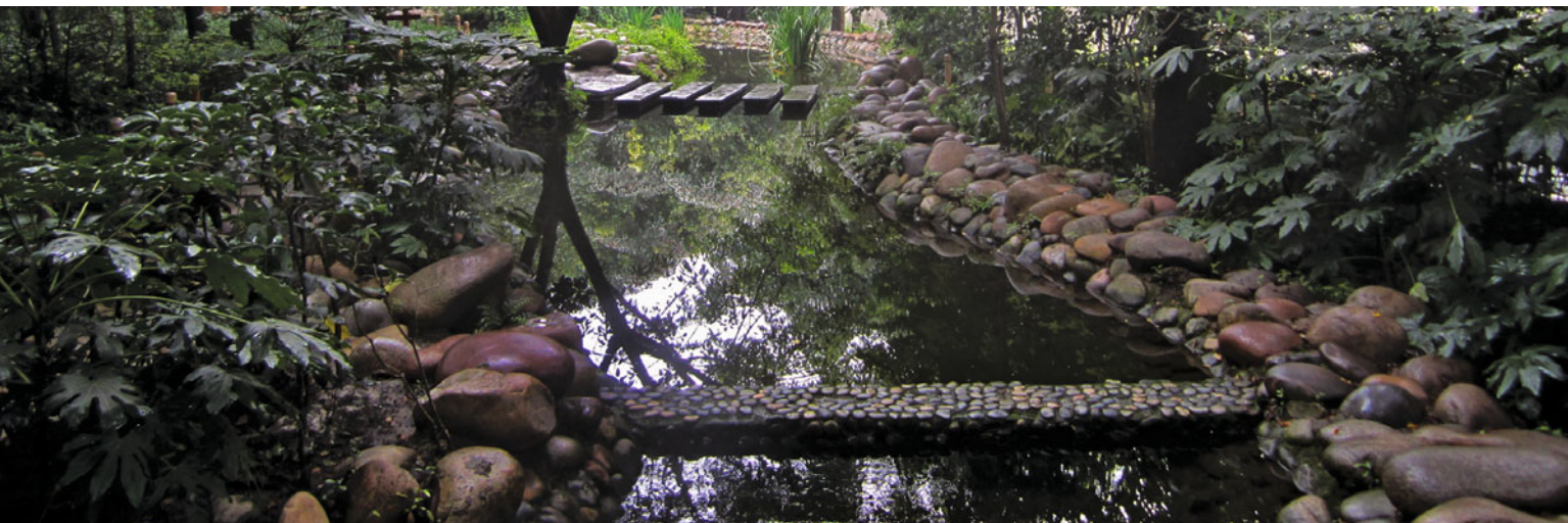
Larger river stones used to retain water edges.
