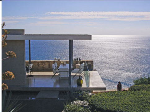
Nearing the edge of the cliff, and the outdoor living room.
