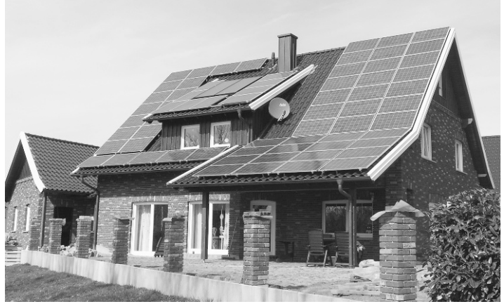
Newly constructed home in Germany with nearly total solar panel coverage.
