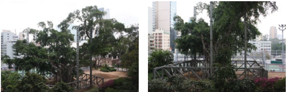
Figure 3.44 Bespoke support system used for a 400-year-old Chinese banyan Ficus microcarpa in Kowloon Park, Hong Kong. Cables fixed to vertical steel pillars support the crown. In turn, a ridged steel framework mounted on piles prevents the heavy structure from damaging the tree roots. Such intensive (and expensive) approaches are only really viable for trees of high cultural or historical importance.
