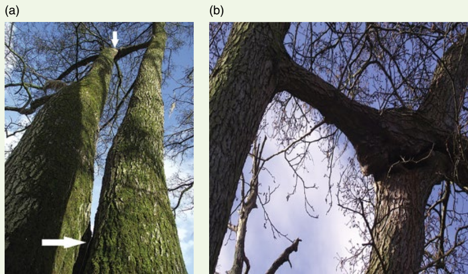
Figure EB3.7 (a) A mature common alder Alnus glutinosa where a lateral branch straddles across the junction between the two main stems of the tree. The lower white arrow identifies the bark-included junction with some minor bulging present, and the upper white arrow identifies the natural brace. (b) The swelling of the branch rubbing against the other stem identifies that this natural brace has been in situ for many years. It would be very foolish to cut away this rubbing branch, despite current industry guidance that encourages this action, for that would make it much more likely that this bark-included junction would fail and half of the tree would fall down in the next strong wind event.
