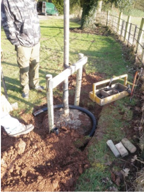
Figure 6.2 (a) An irrigation tube being installed in a tree planting pit. (b) A watering bag placed around a recently planted tree in Copenhagen, Denmark. The bag has a porous base that slowly releases water to the root ball and surrounding soil over a number of hours. This helps reduce surface run-off and ensures deeper soil water recharge. Here, a Treegator® bag is being used, but a number of different brands and designs are available.
