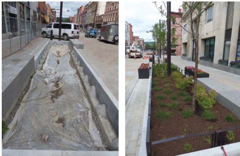
Figure 10.16 Many urban sites, such as these two planting beds in Itacha, New York, USA, provide highly restricted rooting environments for trees. This inevitably leads to water deficits becoming a serious constraint for tree development. When selecting trees for this type of site, choosing a species with a low (more negative) leaf turgor loss point would be valuable as these species are capable of tolerating dry conditions.
