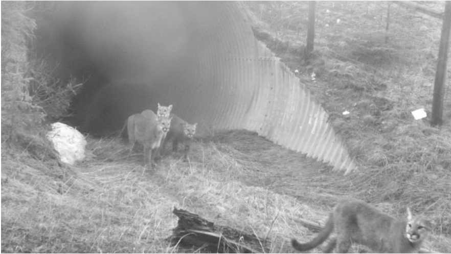
Figure 1.3. Cougars using one of the Banff Wildlife Crossings Project's Bow Valley wildlife underpasses in Banff National Park, Alberta, across Highway 1. (Remote Camera Image, Anthony Clevenger.)
