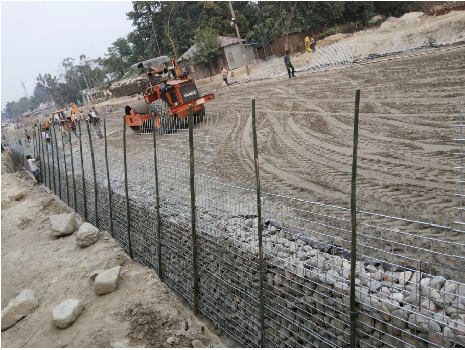
Fig. 8. Compaction of Reinforced Earth fill in progress
