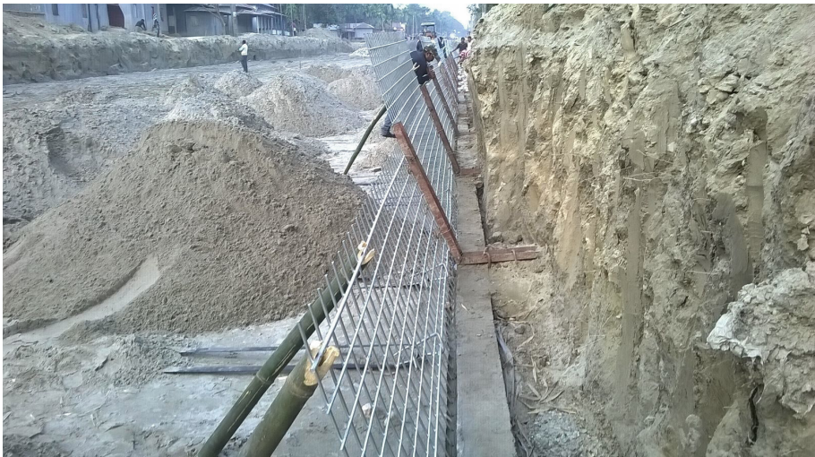
Fig. 5. Erection of first layer of Geotrel
