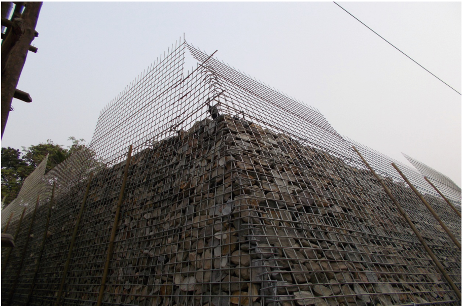
Fig. 7. Erection of Geotrel in progress
