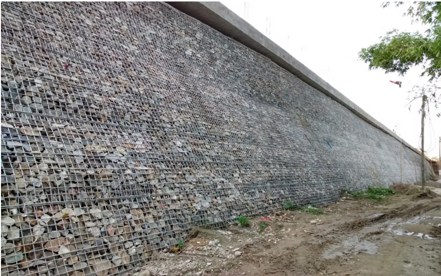
Fig. 9. Construction of Geotrel wall completed
