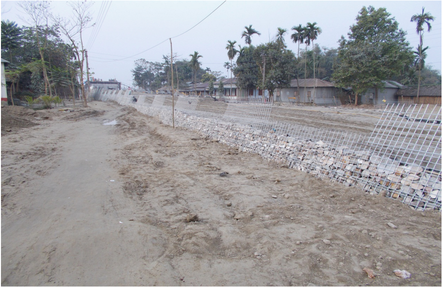
Fig. 6. Erection & boulder filling completed for first layer
