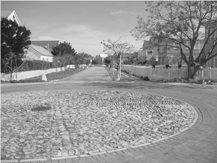
Figure 2-3. Drain inlet and street bioswales, designed by Chris Mulder Associates Inc. to collect storm-water runoff and convey it to a constructed wetland in a residential subdivision. (Source: Michael Murphy.)
