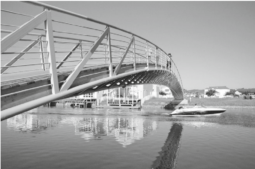
Figure 3-11 Pedestrian bridge at Thesen Islands harbor town, Knysna, South Africa, designed by Chris Mulder Associates Inc./Snyman Roux Structural Engineers, to link residential areas separated by waterways. (Source: Chris Mulder Associates Inc.)
