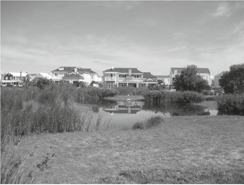
Figure 2-4. Constructed wetland and bird sanctuary for a residential subdivision, designed by Chris Mulder Associates Inc. to treat surface runoff before it enters open waterways. (Source: Michael Murphy.)
