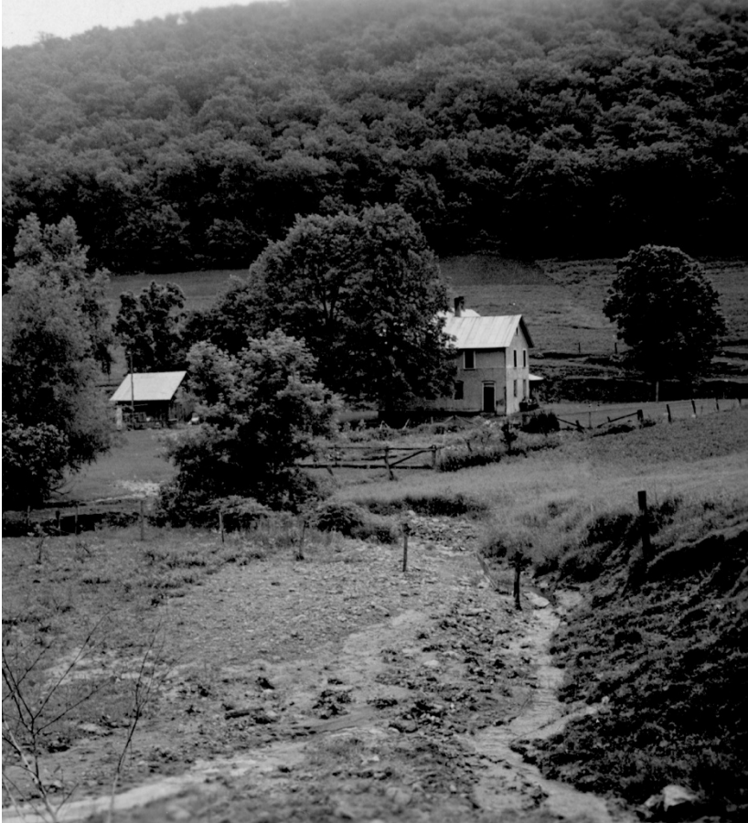
A landowner's livestock grazing on a steep slope broke down the sod and allowed the soil to erode. This caused the formation of a spreading gully that encroached on this neighbor's land.
