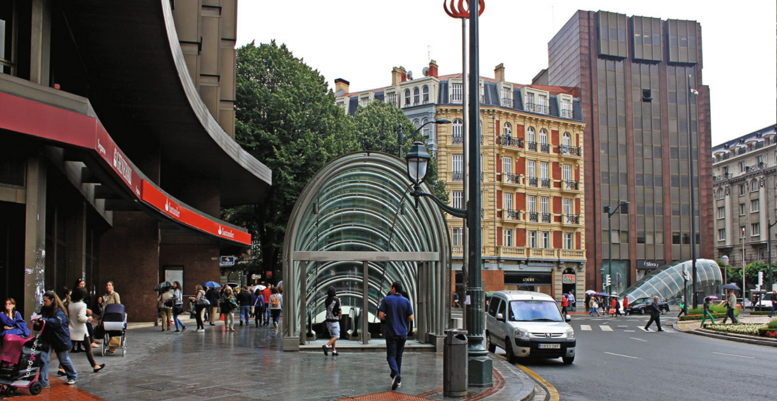
Plaza Moyua, Bilbao (2013). The city's subway, designed by architect Norman Foster, made travel downtown easier and less expensive. (Alexander Garvin)
