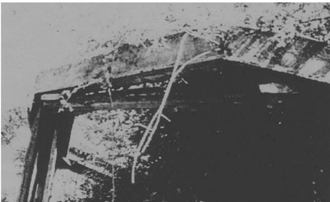
**Fig. 8.7** A view of part of the dome room in 1994 showing the horizontal wall plate and directly above it the octagonal base-ring of the dome (*Photograph Gary Wilmhurst*)
