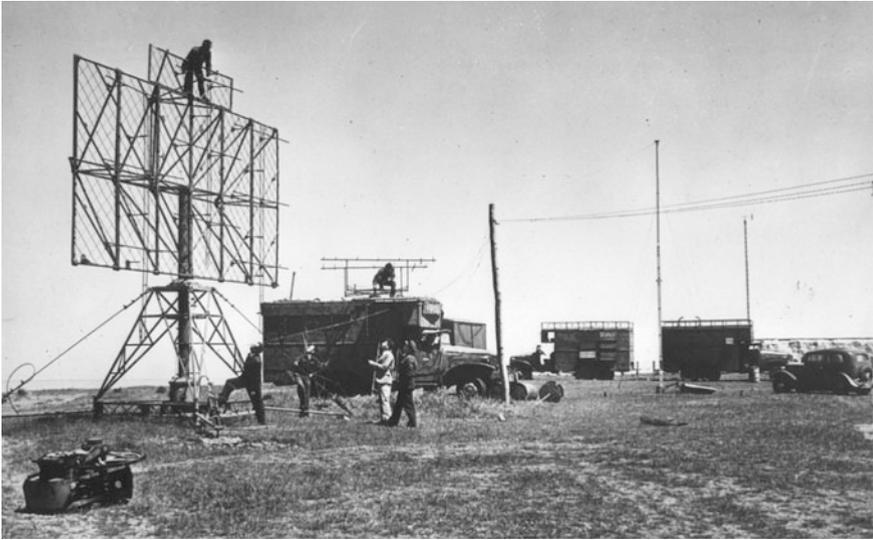
**Fig. 23.9** Installation of the ‘Canterbury Project’ 97.5 MHz radar antenna at Wakanui Beach near Ashburton. In the background are associated equipment trucks (Orchiston collection)
