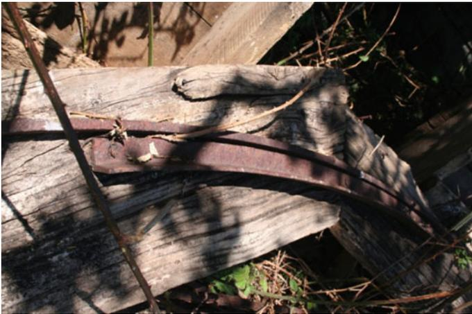
**Fig. 8.12** A collapsed section of the horizontal wall plate with the U-shaped channel, in 2014 (*Photograph* Gordon Hudson)
