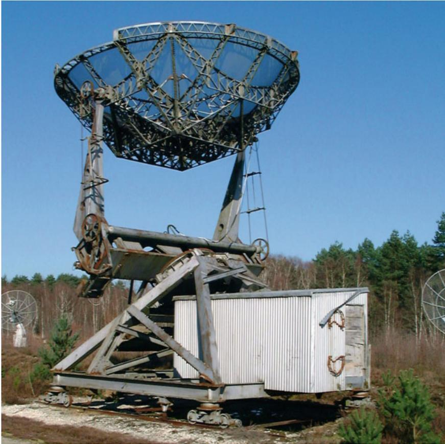
**Fig. 1.19** A recent photograph of the sole surviving Würzburg antenna at the Nançay Radio Astronomy Field Station in France. Originally there were two of these dishes, mounted on rails, and they operated as an interferometer. They were used, mainly, to measure the angular sizes and structure of discrete radio sources (see Orchiston et al. [2007](#))
