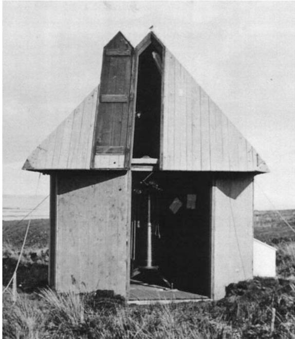
**Fig. 14.13** View of the Chatham Islands 'Transit House' with a wall removed, showing the broken tube transit telescope and its brick pier (*Courtesy Alexander Turnbull Library, Wellington, Ref. PAColl-0058-03*)
