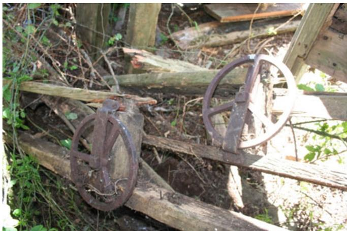
**Fig. 8.13** Collapsed sections of the octagonal base-ring of the dome, showing the wheels, in 2014 (*Photograph* Gordon Hudson)
