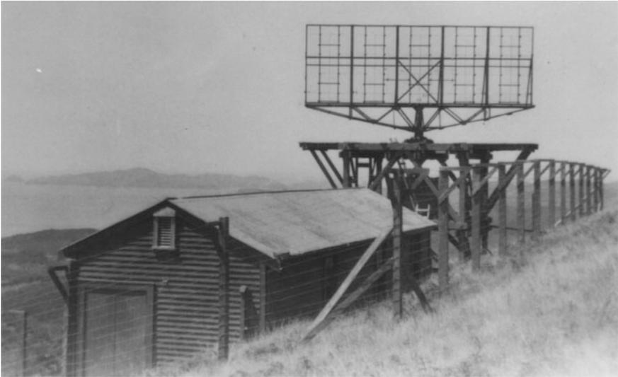
**Fig. 23.5** The Whangaroa radar station, showing the 200 MHz broad-side array and associated technical building (Orchiston collection)
