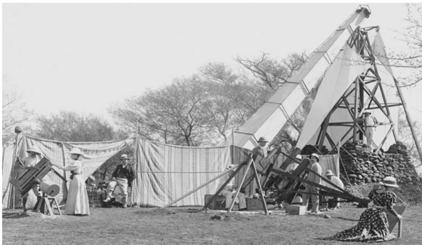
**Fig. 1.23** A scene showing the Lick Observatory party ready to observe the 22 January 1898 total solar eclipse from Jeer, India. All of the instruments are in place and the volunteers are at their practice stations. The 40-ft Schaeberle Camera with its twin wooden towers dominates the scene (after Orchiston and Pearson 2011: 199)
