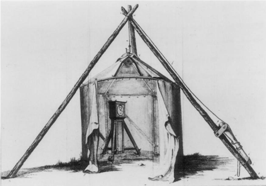
**Fig. 5.13** The type of tent observatory used by the Second Voyage astronomers (after Wales and Bayly 1777: Plate II)
