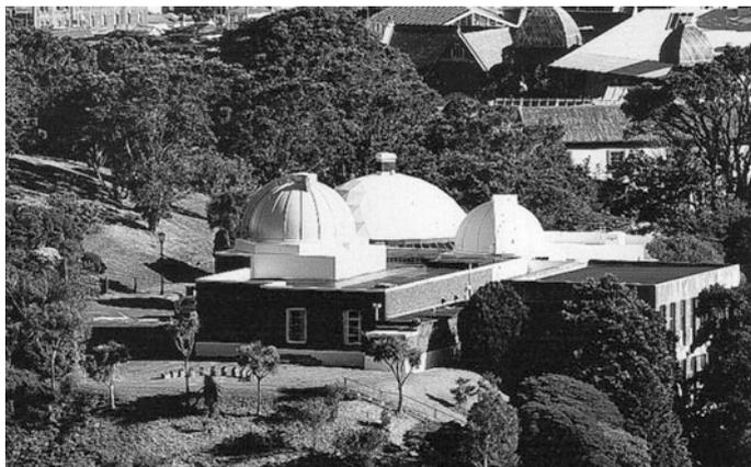
**Fig. 13.14** Carter Observatory in the late 1990s. The Cooke telescope is in the foreground left-hand dome. In the small right-hand dome, also part of the original building, is a 41-cm Boller & Chivens reflector, while the large dome at the rear, added at the end of 1991, houses a planetarium. The two-storey library-office wing on the extreme right was constructed during the 1960s (Orchiston collection)
