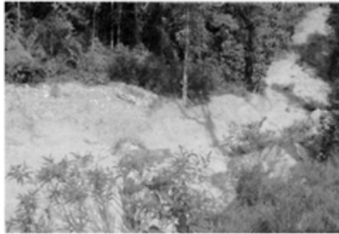
Figure 5.67. Travel of debris and failed mass downhill.
