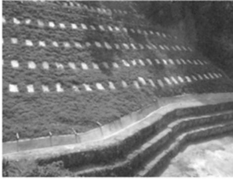
Figure 5.65. Completed soil nailed slope.
