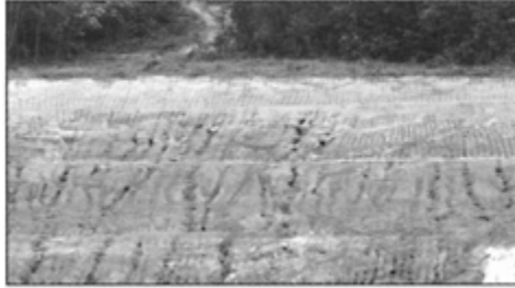
Figure 7.5. Rills and gullies on slopes.
