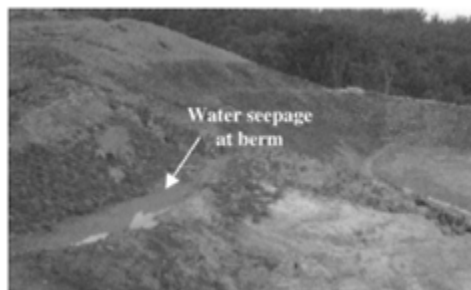
Figure 5.19. Water seepage at berm.
