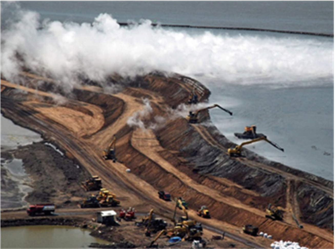
Fig. 23 Maintenance of dykes
