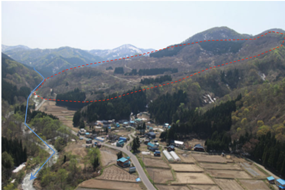
Fig. 5 Full view of the Tozawa landslide site
