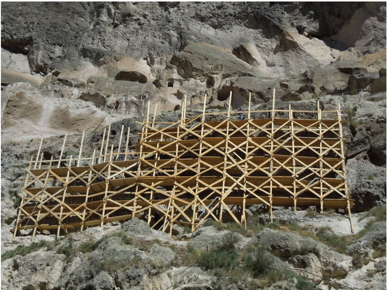
Fig. 30 The wood scaffolding realised in Vardzia
