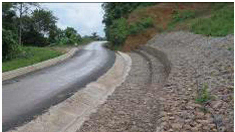
Fig. 5 Resilient landslide protection measures in Bountai District (Lao PDR) provided communities with safer access to public services
