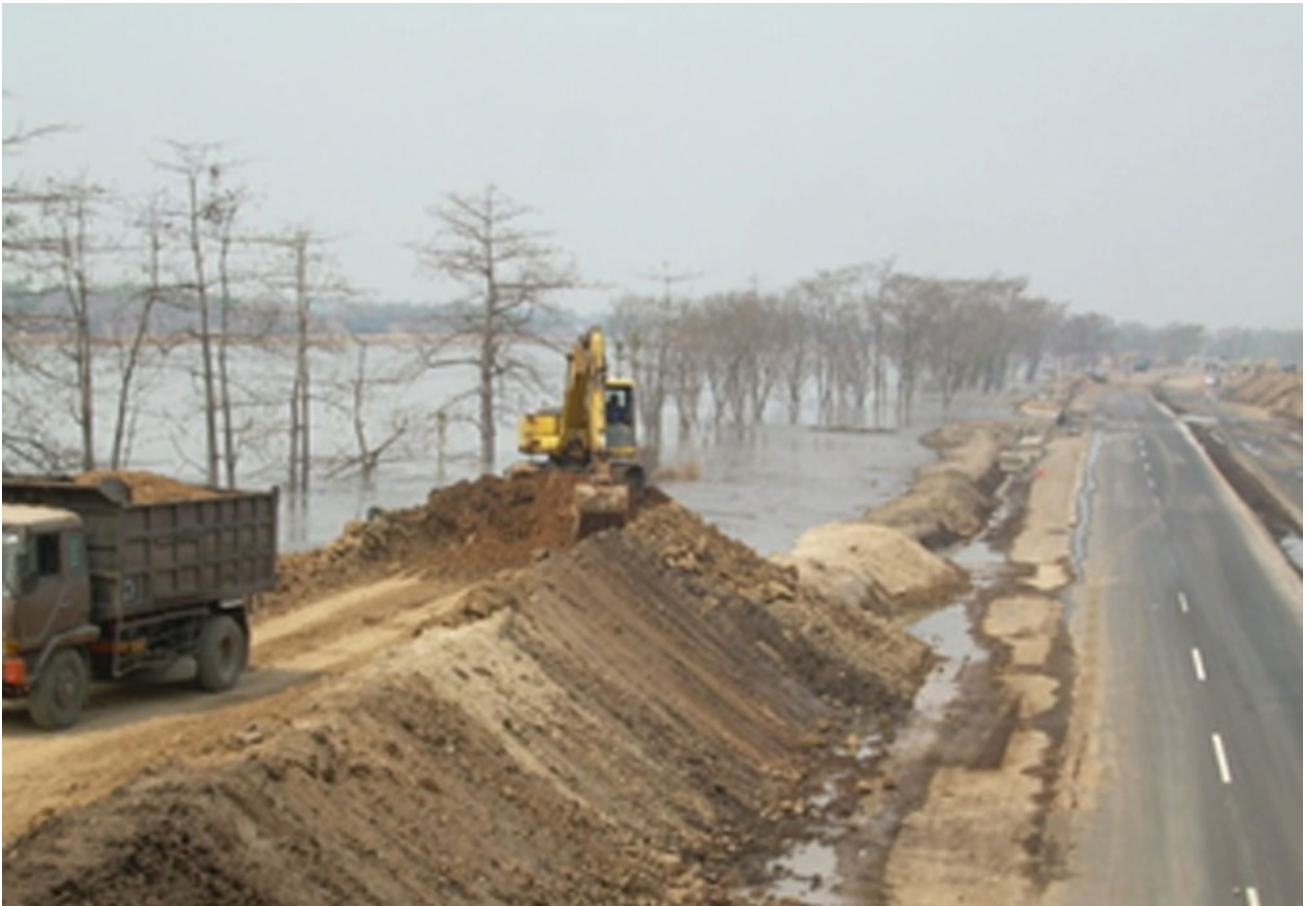
Fig. 21 Construction of permanent dykes (BPLS 2007)
