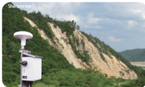
Shamen-net Shamen-net is a total monitoring system integrating GPS and other monitoring devices (Measurement precision: +/-1mm, on a real time basis)
