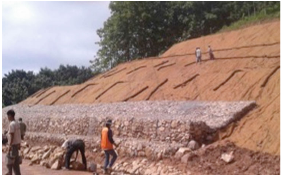
Fig. 7 Landslide mitigation, Lao PDR
