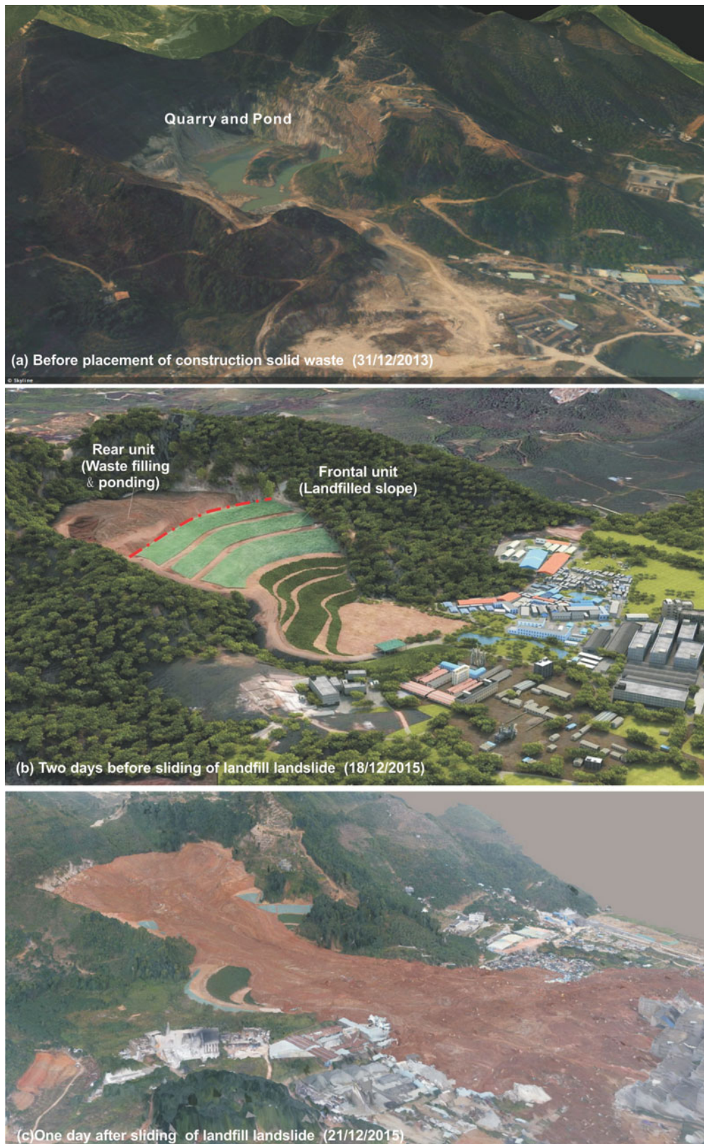
Fig. 9 Comparison of images showing the Hong'ao Village location, landfill, and landslide. a Remote-sensing image taken in December, 2013 (three months prior to CSW placement); b remote-sensing-based image taken on December 18, 2015 (two days before the landslide); and c aerial view taken on December 21, 2015 (one day after the landslide) from a UAV
