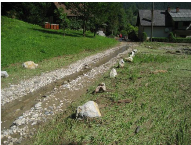
Fig. 7 The consequences of flooding it’s clearly visible; the torrent diverted from original channel and took the forest road as its riverbed (Kambič 2009)
