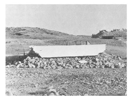
**PHOTO 24.3** Serdo's school, which had a heavy cement-slab roof, was completely flattened by the earthquake. Fortunately the students were not in school at the time. A new school, more appropriately constructed, has since been built on the same site (1969). Photo modified from Gouin (1979) and used by permission of the International Development Research Centre, Ottawa, Canada
