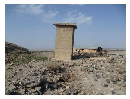
**PHOTO 24.4** Serdo's concrete water tower was tilted about  $5^{\circ}$  to the southwest by the earthquake, and much of its brick facing fell off. It remained standing, still tilted at this angle, until at least 2013. I have heard that it has since been demolished (2011)
