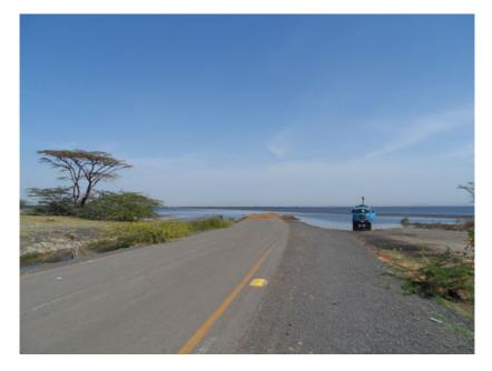
**PHOTO 19.11** The end of the road! The water of Lake Besaka has risen so high that the road cannot be raised any further, and has had, together with the railway line, to be diverted to the north (2013)
