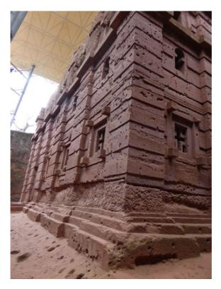
**PHOTO 14.7** Damage by water seepage to the base of Bet Emmanuel. The cover erected over the top of the church, of which a portion can be seen, has not addressed this problem. The Italians attempted to repair the damage with cement, which has now been removed (2014)
