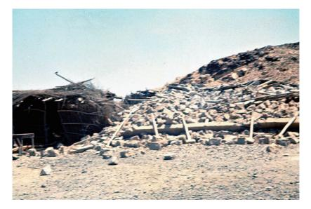
**PHOTO 24.2** Another photo taken two weeks after the first shock struck Serdo. Notice on this photograph, and on PHOTO 24.1, that the structures made of sticks, wood, or corrugated iron remained standing while those of bricks, concrete and with heavy roofs collapsed (1969)
