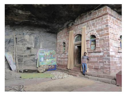
**PHOTO 14.10** The monastery of Nakuta La'ab, built of bricks of tuff within a basalt cave. Water drips through the roof into the church and is collected in basins crafted from basalt (2014)
