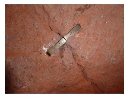
**PHOTO 14.6** A crack in the wall of Bet Raphael. The marker was placed across the crack in 1968 to monitor the rate of widening. Between then and 2014 it has widened by about 2 mm (2014)
