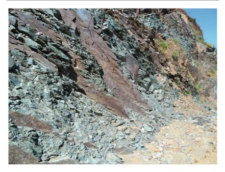
**PHOTO 9.10** Slate in road cutting on the southern side of the Takeze River. The slate easily breaks along its cleavage planes and slides onto the road. If you look carefully you can see a geological hammer for scale (2014)
