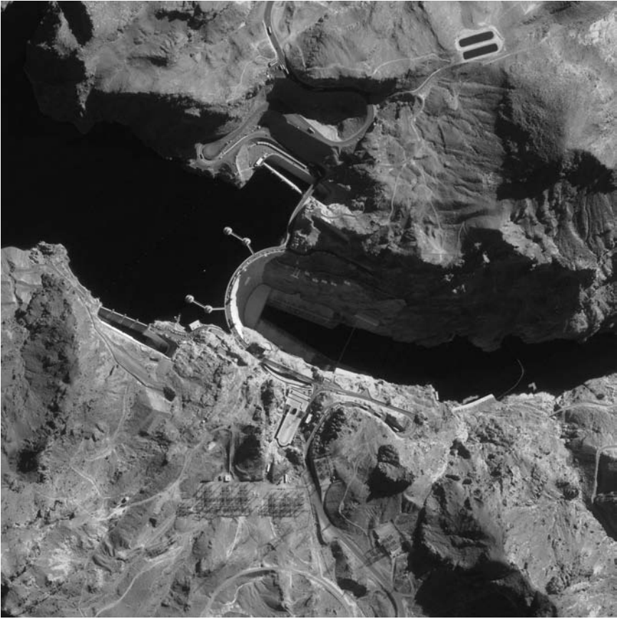
Figure CS4.3 Hoover Dam: December 25, 1999. 1-m resolution image from IKONOS. (From Space Imaging Corporation. With permission.)
