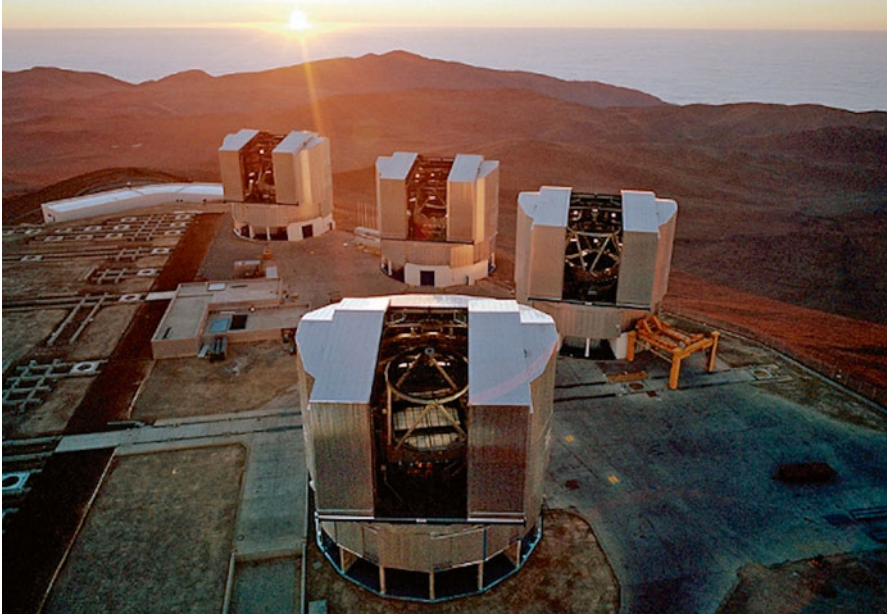
Fig. 6.10 The Very Large Telescope of the European Southern Observatory on mountain Paranal in Northern Chile. It consists of four telescopes with primary mirrors of 8.2 m diameter. Together, when the light of the four telescopes is combined, they form the largest optical telescope of the world, with an effective diameter of 16.4 m
