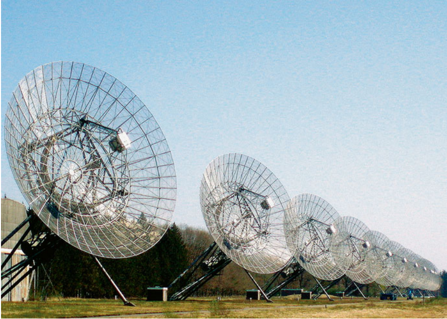
Fig. 4.15 The Westerbork Synthesis Radio Telescope (WSRT) was inaugurated in 1970. It consists of 10 fixed-location and four movable dishes of 25 m diameter each, stretched along a baseline of 3 km (about 2 mi.). Although since 1980 larger radio arrays have been constructed in the USA and India, in certain wavelength ranges the WSRT still is the most sensitive radio telescope in the world
