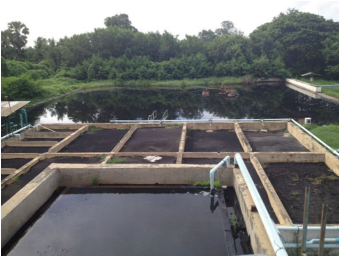
Fig. 6 Solar evaporation plant used in small-scale textile coloration units in Tirupur, India
