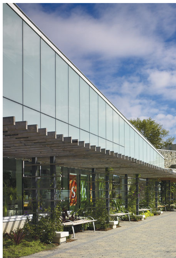
« Above the trellis, fritted glass filters and diffuses sunlight, creating an indoor space that is bright while minimizing glare and heat gain.
