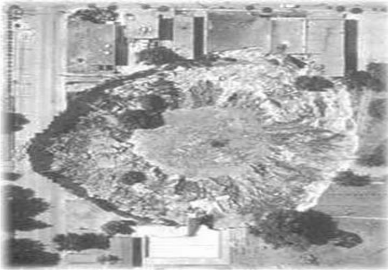
Fig. 5.1 View of a sinkhole swallowing a house in Central Florida
