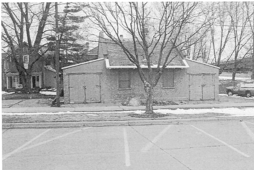
Figure 4. Residential garage. Sanborn maps show an UST where the left-hand garage doors now exist.
