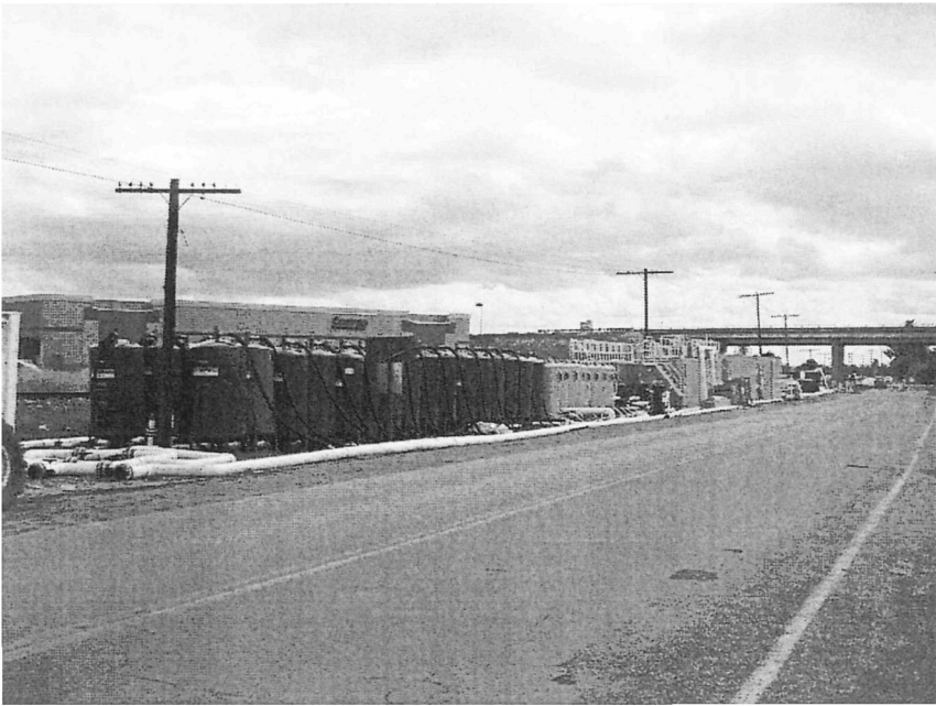
Figure 5. Complete Filtration System
