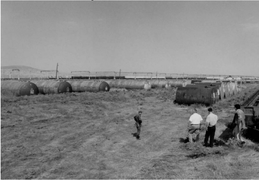
Photograph 5 , Storage of Samine rocket fuel in tanks similar to those used for the storage of the oxidizer at the Alyat depot. The tanks are lying on the bare ground. A strong characteristic amine odour surrounds the storage site.
