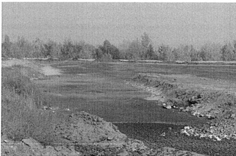
Fig 3. Surface covering in progress at the disposal site
