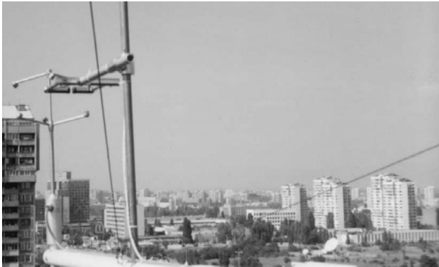
Figure 8: The meteorological tower at the National Institute of Meteorology and Hydrology (NIMH) in Sofia, sonic anemometers were mounted near the platforms (upper panel) and a view from the tower to the west (lower panel) with a sonic anemometer in the foreground.
