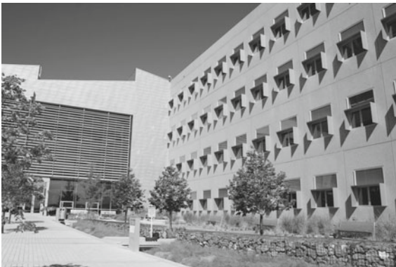
NREL Research Support Facility wall detail. (Bill Gillies.)
