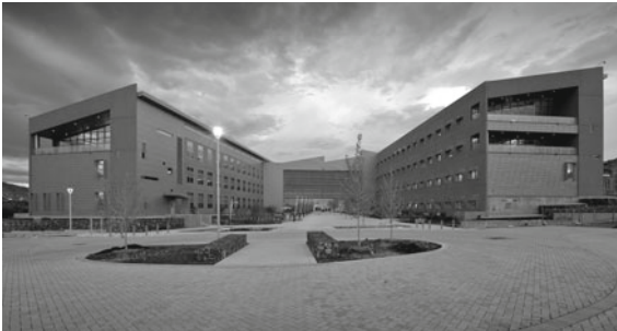
NREL Research Support Facility, two building wings with entrance. (Dennis Schroeder, NREL.)
