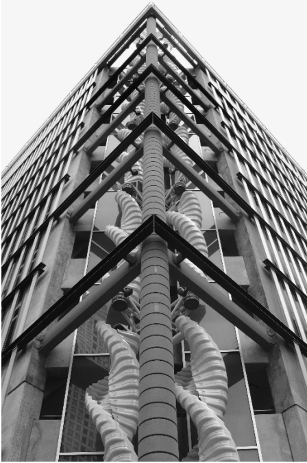
Urban wind turbines on a parking garage in Chicago provide power for the building's exterior lighting.
