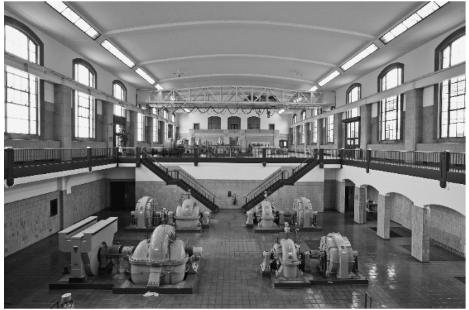
The R. C. Harris Water Treatment Plant in Toronto opened in 1941.
