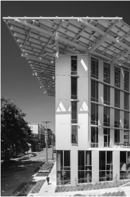
The Bullitt Center in Seattle is considered one of the greenest commercial buildings in the world.
