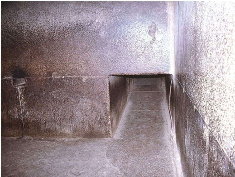
Fig. 6.10 Giza. Detail of the King's Chamber in Khufu pyramid, completely built with huge granite blocks. On the right of the entrance (north) the mouth of the northern upper channel can be seen
