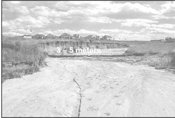
Figure 1. Example of an eroded waterway in response to upstream urbanisation Photograph by permission of the Urban Drainage and Flood Control District.
