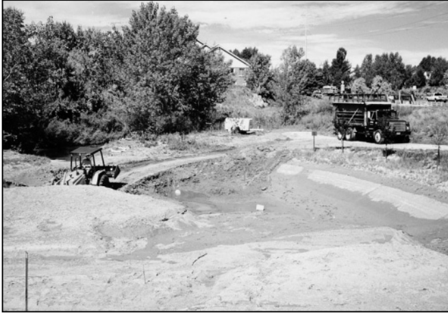
Figure 4. Sedimentation pond during a cleaning operation. Photograph by permission of Urban Drainage and Flood Control District
