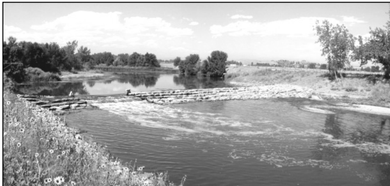
Figure 9. A 1.2 m high grouted boulder grade control structure at the Henderson flow measuring gauge site; safe for boaters and permits fish migration.
