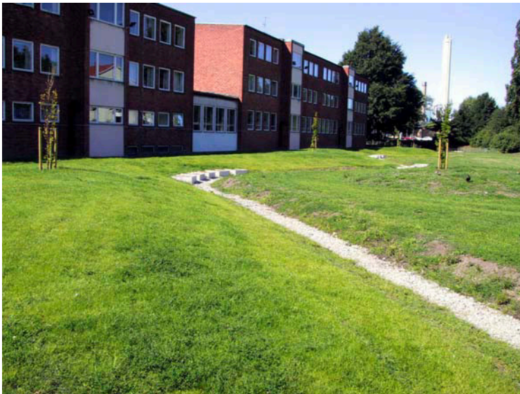
Figure 7. Open drainage ditch in the existing park in Augustenborg
