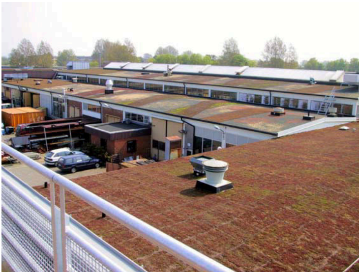
Figure 6. A section of the green roof installation at Augustenborg in Malmö.
