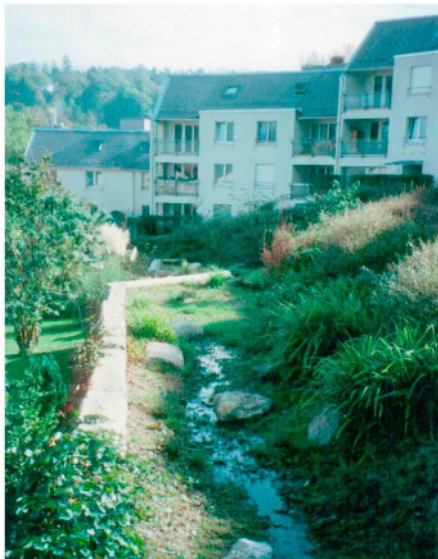
Fig. 12. The day-lighted stream has been integrated into the landscaping of a new residential area.
