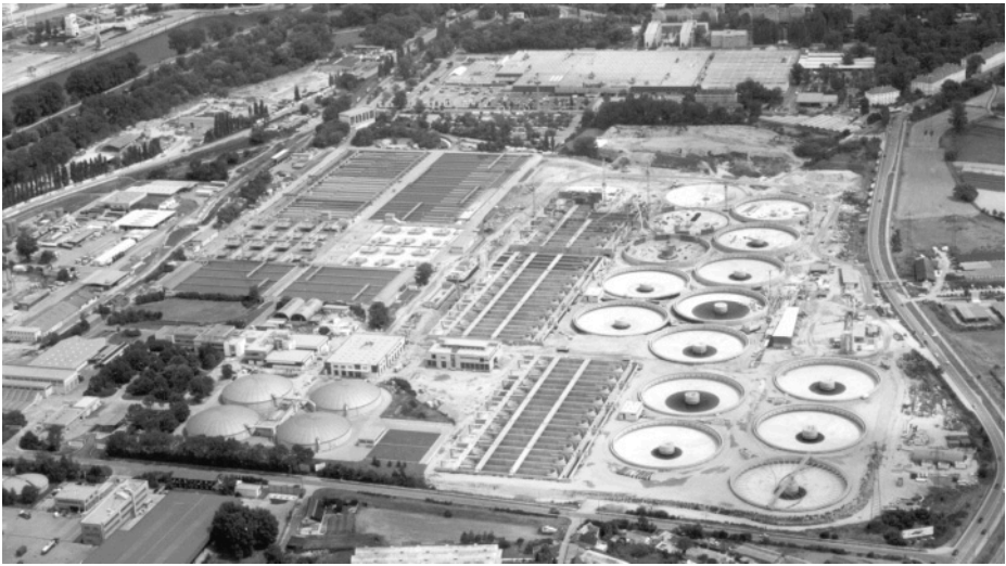
Figure 5: Construction phase of MTPV in July 2003
