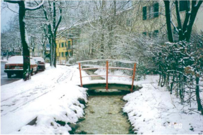
Fig. 5. Along the "in der Ey"- Street, despite the narrow space, it was possible to build the day-lighted stream between the sidewalks and the private properties.
