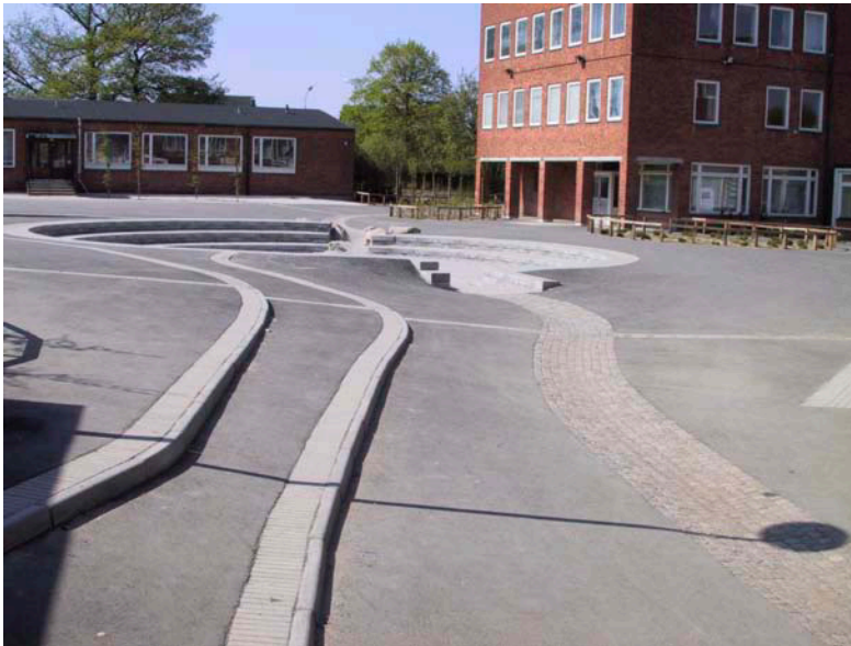
Figure 8. Detention basin in the form of an amphitheatre in the schoolyard of Augustenborg
