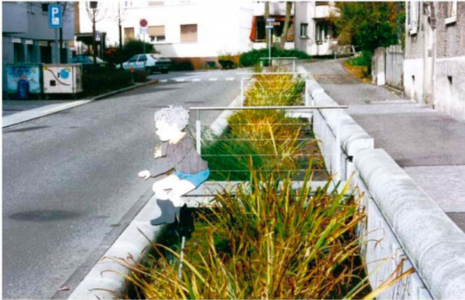
Fig. 13. The day-lighted Nebelbach brook forms part of the public street.
