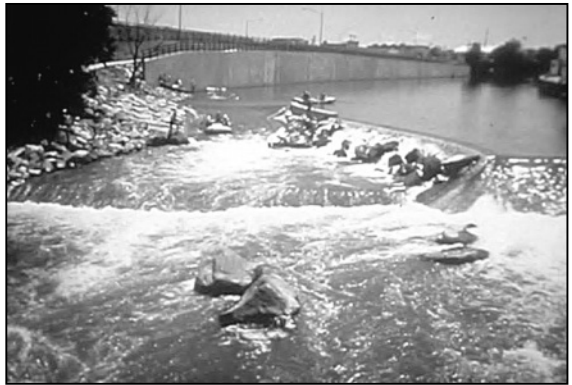
Figure 11. A 2-meter high “killer drop” modified to include a boat chute. Note the strong “keeper” in “before” and the strong central “jetting” current “after” pictures. Photograph by permission of Urban Drainage and Flood Control District.
