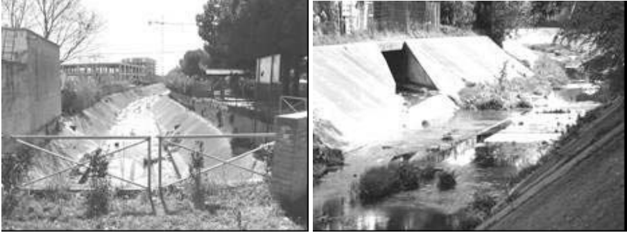
Figure 2. Channelised and confined stream in a heavily urbanised area (left) and sewer outfalls (right)
