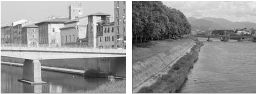
Figure 3. Concrete bank protection (right) and concrete toe protection of delimiting wall in an urban river (left)
