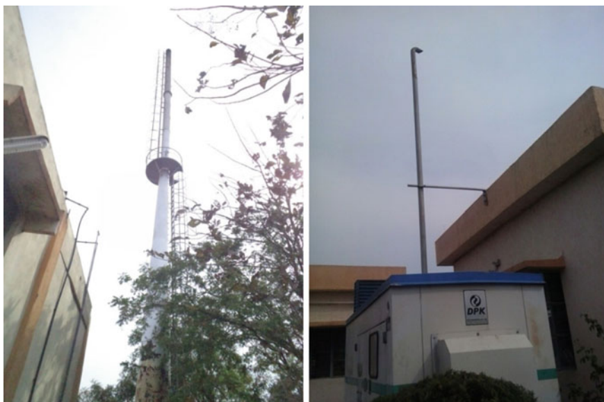
Fig. 4.7 Examples of chimneys without bend and with bend. Bend in later location is provided to avoid entry of rain water
