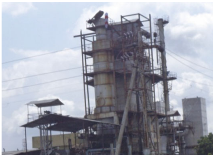
Fig. 1.21 Corroded steel structure
