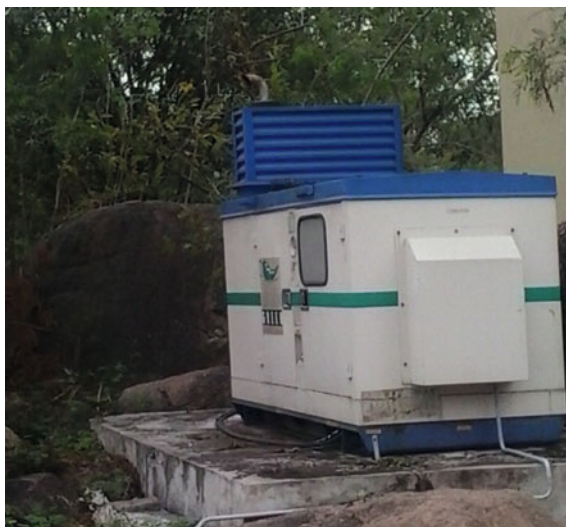
Fig. 4.5 Example of wrong practice—diesel generator next to building with exhaust not attached to tall chimney
