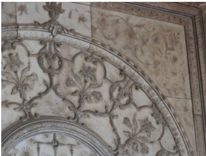
Fig. 1.17 Intricate carvings being washed away due to air pollution
