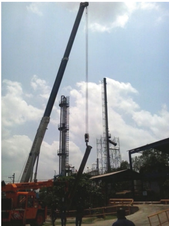
Fig. 9.3 Erecting chimney using crane
