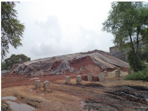
Fig. 5.16 Cloth covered on soil to control air pollution
