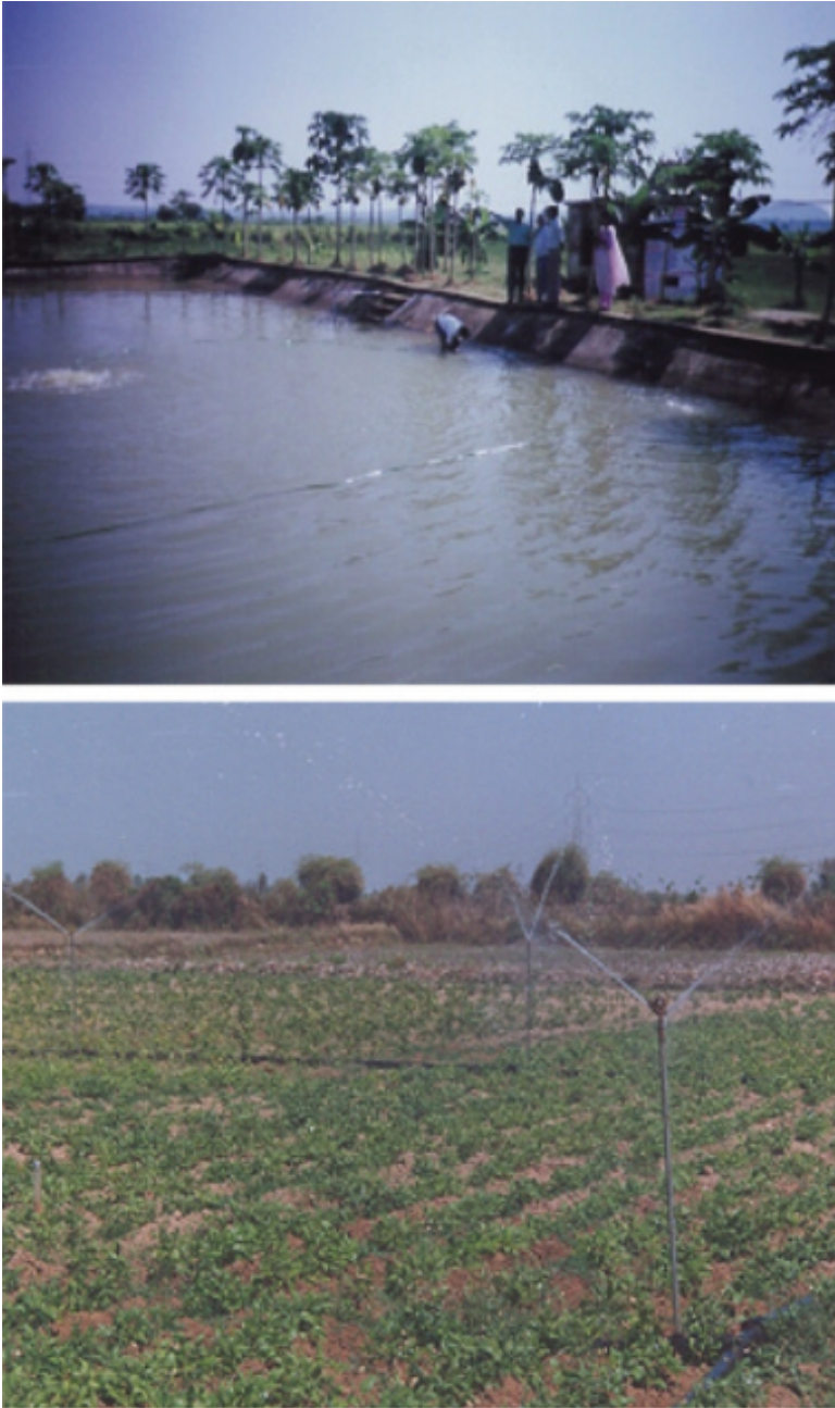
FIGURE 16.2. View of the adjunct reservoir along with pump house (top); View of sprinkler irrigated potato in the command area (bottom).
