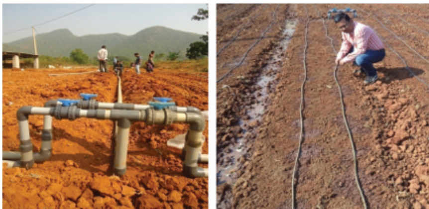
FIGURE 8.3 Installation of drip irrigation (left) and laying of laterals on the raised bed (right).
