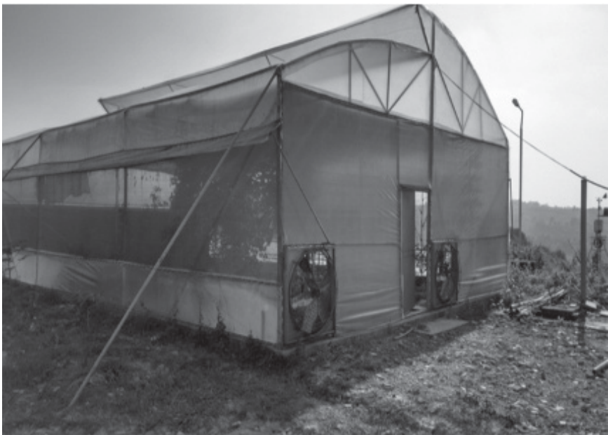
FIGURE 2.2 View of a greenhouse structure selected for experiment in the study site.
