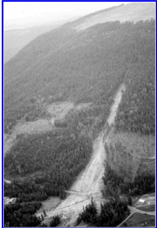
Figure 8. Debris flow at Philpott Road, B.C.
