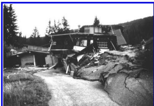
Figure 13. The restaurant was destroyed at the end of July, 1994, due to a shear movement.
