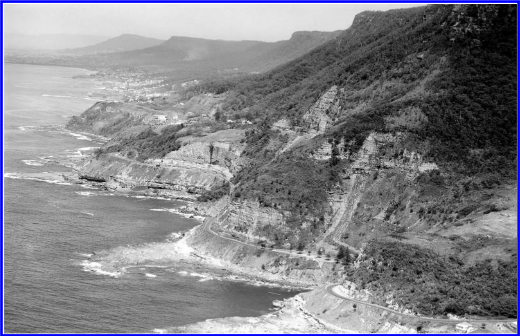
Figure 3. 1967 aerial photograph looking south at Lawrence Hargrave Drive (near the base of the escarpment). The geological units which make up the escarpment are shown on Figure 4. The Bulgo sandstone (centre right of photo) only forms cliffs in the project area (foreground) where the escarpment has been oversteepened by coastal erosion. In the distance there is a mature escarpment with a coastal plain. Other features described by Hendricks et al. (in prep.). Photo courtesy of RTA photo archive.
