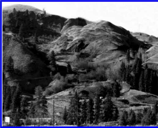
Figure 1. The Pollock Landslide complex in central Idaho.
