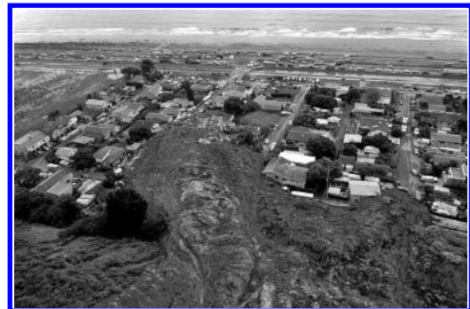
(a) Post-landslide looking seaward.
