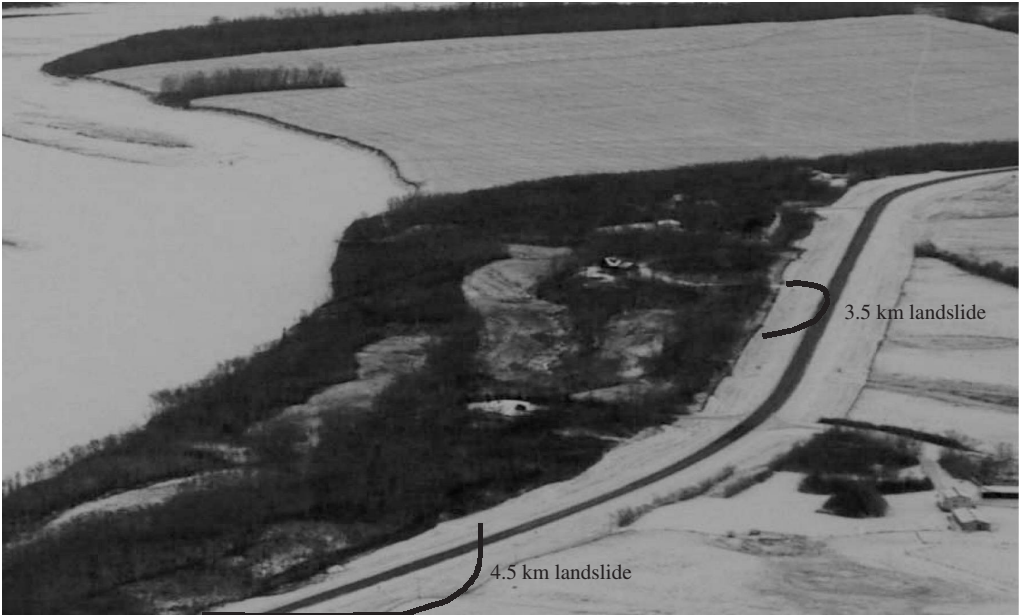
Figure 8. Prince Albert Highway 302 landslide extents. Landslide at bottom left is 4.5 km from penitentiary.
