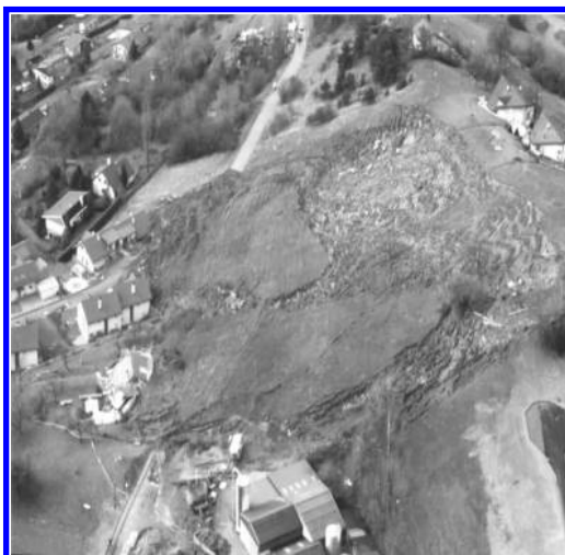
Figure 15. Three houses were destroyed in 1990 in the upper part of the Commune of Belmont s/Lausanne, which induced the local authorities to proceed to a complete inventory of landslides.
