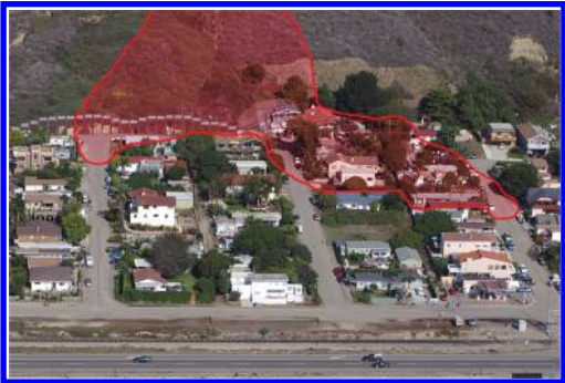
(b) Pre-landslide looking landward with outline of landslide debris
