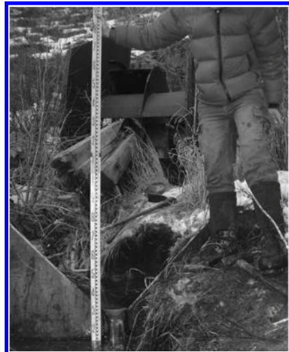
Figure 14. Outflow weir installed at the Frank Mine entrance.
