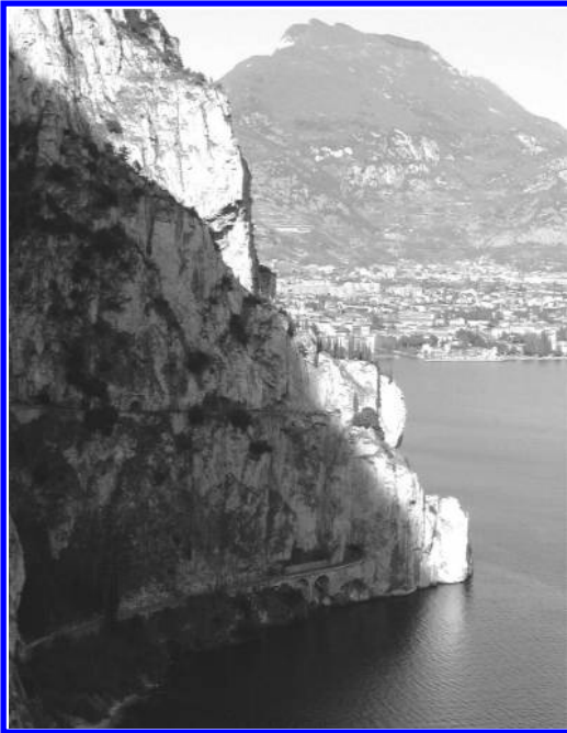
Figure 13. Two-lane roadway at base of 1000 m high cliffs in Italy (note road and tunnel at base of cliff).
