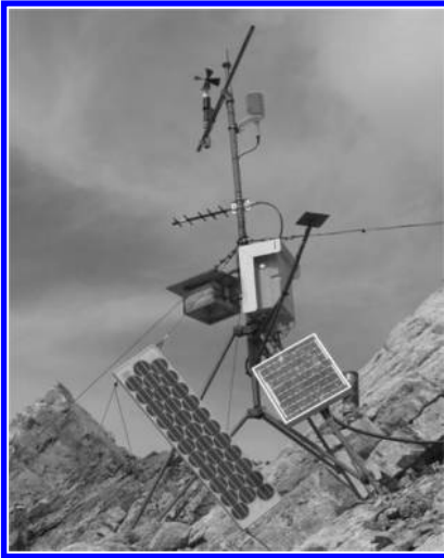
Figure 13. Refurbished weather station on the west side of South Peak.
