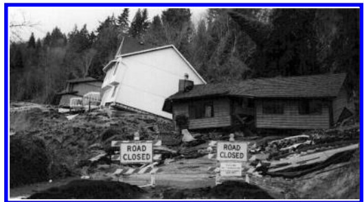
Figure 6. Property damage on large slow moving landslide in Kelso WA (by NW Geoscience).
