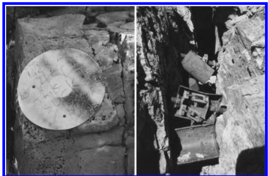
Figure 7. Defaced photogrammetry target (left) and vandalized Moiré crack gauges (right) observed in 1999.
