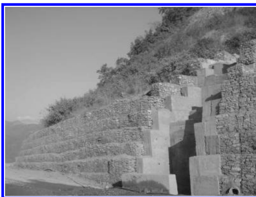
Figure 10. Krishna-Bhir landslide in 2004 November after stabilization by countermeasures.
