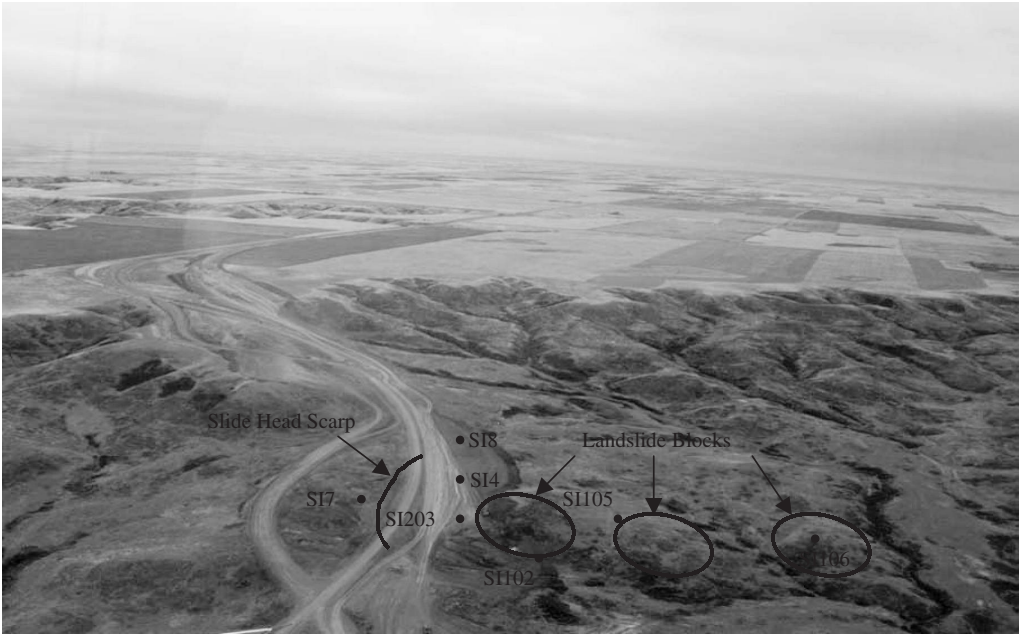
Figure 4. Approximate location of landslide and slope inclinometers at Frenchman River Valley.
