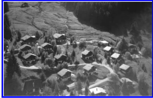
Figure 12. View of the village of Falli Hölli at the beginning of the crisis. These houses moved over more than 200 m. Some drainage ditches are seen in the back of the village.
