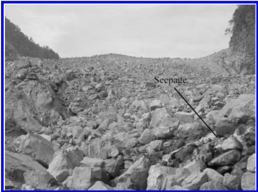
Figure 3. Downstream face of the Tsatichuu deposit with seep point. The face failed catastrophically after seep progression in combination with heavy rainfall (photo C. Massey).
