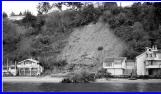
Figure 7. Casualties (four fatalities) and property damage due to landslide in Bainbridge WA 1997 (by WSDOE).
