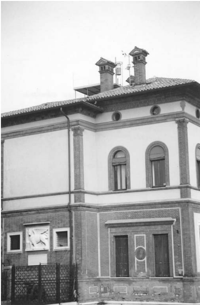
Figure 7 In urban and suburban areas, the only available sites for rain gauges may be on rooftops as shown in the picture. A color version of this image is available at http://www.mrw.interscience.wiley.com/ehs
