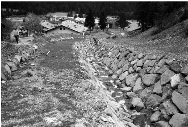
Figure 6 Artificial channel on Torrent Gola – Trentino Italy (Provincia Autonoma di Trento, 1991). A color version of this image is available at http://www.mrw.interscience.wiley.com/ehs
