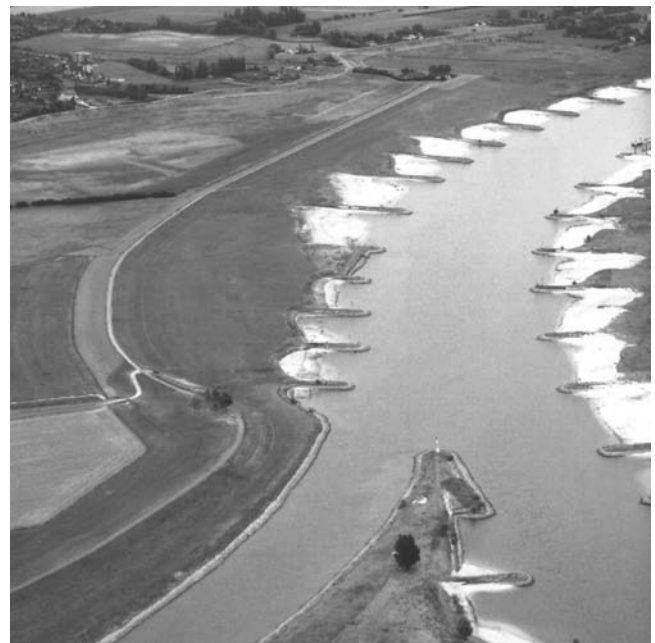
Figure 9 The morphological state of groyne fields is influenced by navigation (flow from top to bottom). A color version of this image is available at http://www.mrw.interscience.wiley.com/ehs
