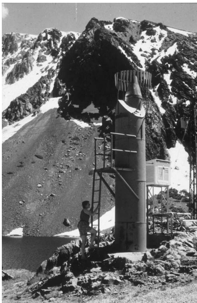
Figure 8 In areas of heavy snowfall, gauges may have to be mounted on towers above. A color version of this image is available at http://www.mrw.interscience.wiley.com/ehs
