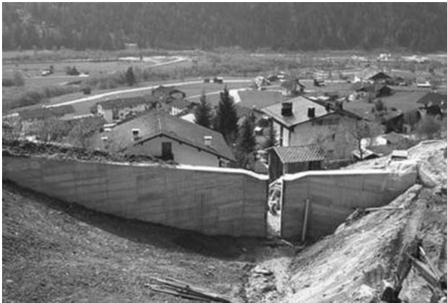
Figure 8 Slit dam on Rio Inguela, Trentino Italy (Provincia Autonoma di Trento, 2002). A color version of this image is available at http://www.mrw.interscience.wiley.com/ehs
