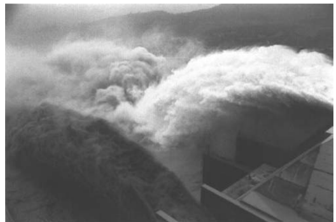
Figure 3 Combined release of clean (white) and heavily sediment-laden (dark) water through the Xiaolangdi Dam, Yellow River, China. A color version of this image is available at http://www.mrw.interscience.wiley.com/ehs
