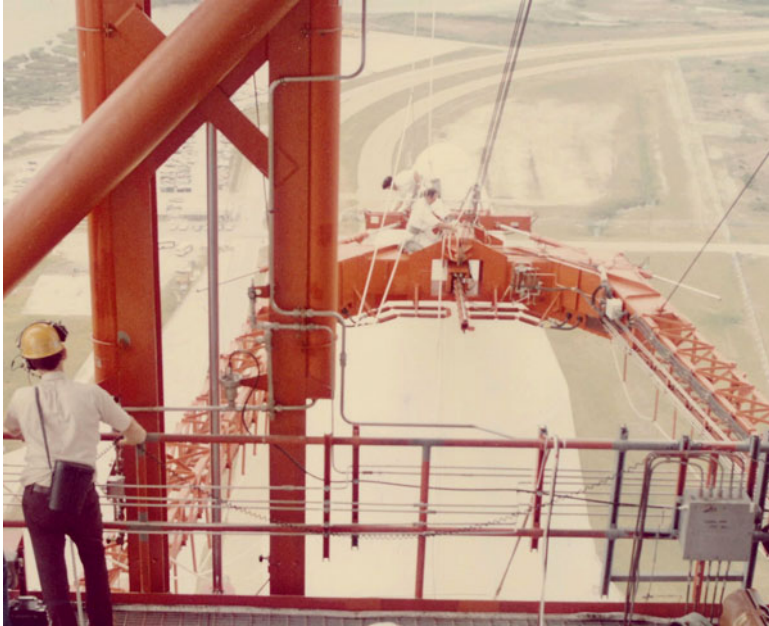
8.4 Nerves of steel: Boeing workers at the end of the viscous damper system, at the nose of the Skylab Orbital Workshop. They are about 400 ft (122 m) above the ground, without a safety net. Source: NASA/Ward
