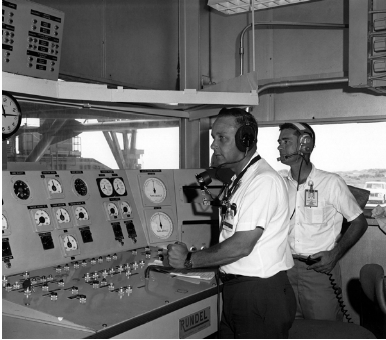
2.12 Harold Pyles ( right ) monitors operations in the control room of the LC-37 service structure. The structure moved between pads A and B on rails. Source: NASA/Ward
