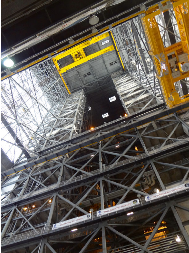
5.12 Author's photo from November 2011 showing the relationship of the transfer aisle crane (right) and a high bay crane. The "diaphragm" (opening) into high bay 3 is clearly visible. To provide a sense of scale, the low end of the diaphragm is 165 ft (50 m) above where the author was standing on the VAB floor. Source: Ward
