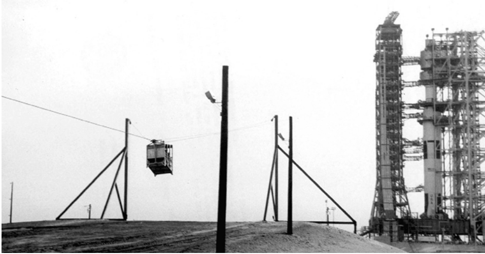
8.28 To slow the gondola at the end of the slide wire run, the support system leveled off the wires and then raised them slightly. In the Shuttle-era system, drag chains slowed the escape baskets, which then hit a net. Source: NASA/Ward
