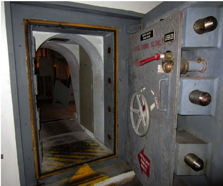
8.23 Door to the pad A blast room, similar to doors used in missile silos (Photo by the author, August 2013). Source: Ward
