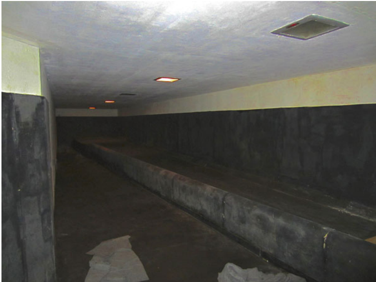
8.22 The deceleration ramp in the rubber room. A slight upward slope was supposed to be sufficient to slow people down, but it was still dangerous (Photo by the author, August 2013). Source: Ward
