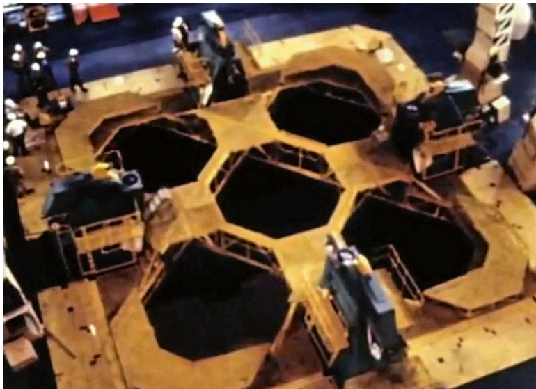
5.28 The S-IC engine servicing platform was installed in the LUT before the S-IC stage was erected. The platform was removed before rollout by lowering it through the LUT's flame compartment. Source: NASA/Ward
