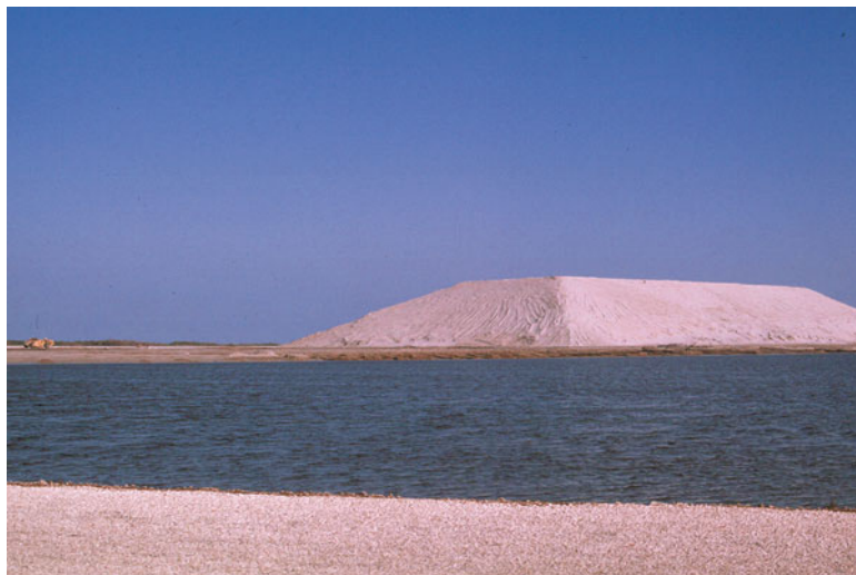
7.9 A mound of dredged material piled atop the pad A site, October 1964. The weight of this pile of material compacted the soil on which the launch pad would be constructed (Photo courtesy Frank Penovich). Source: Penovich
