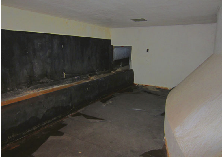
8.21 The exit from the escape chute that came down through the pad structure into the rubber room. The outer wall of the blast room is at right (Photo by the author, August 2013). Source: Ward
