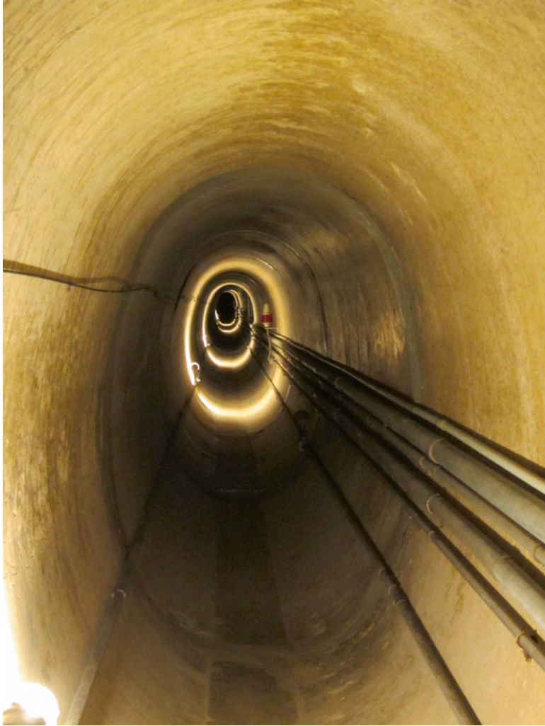
8.25 Ventilation tunnel leading from the blast room to an air intake building at the perimeter of the pad (Photo by the author, August 2013). Source: Ward
