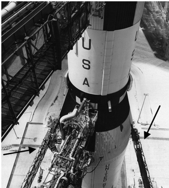
5.21 S-II/S-IVB damper system in use on AS-500F at the launch pad. The dampers are the two thinner arms at center (arrowed). Source: NASA/Ward
