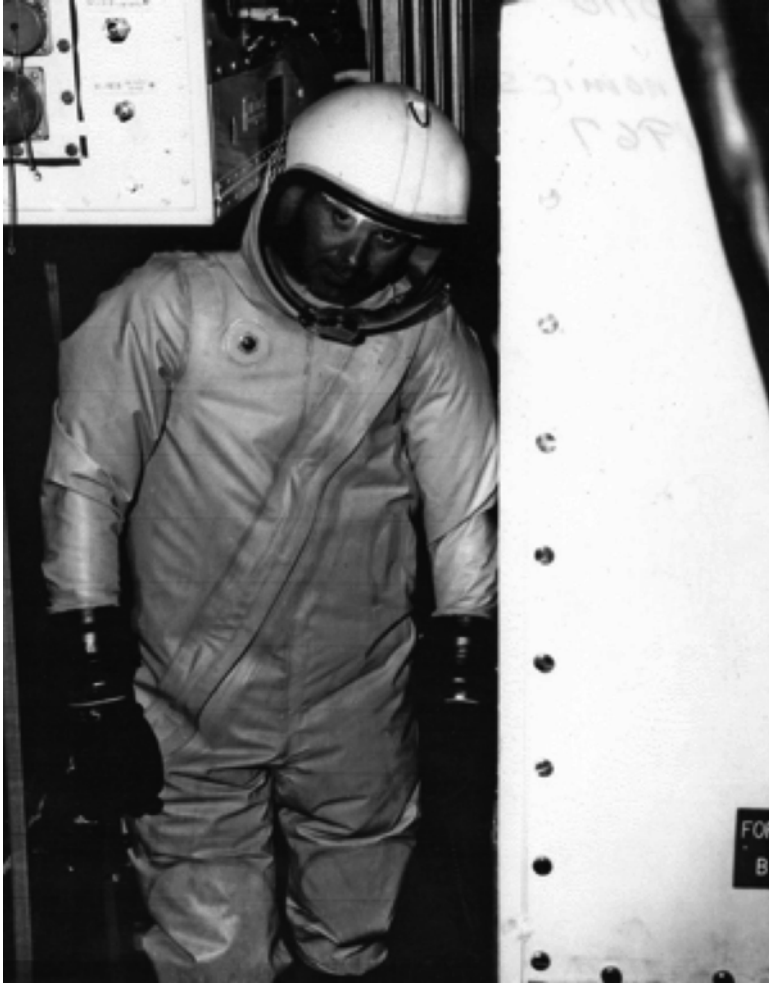
8.9 SCAPE suit for hypergolic loading operations, 1967 (Courtesy of John Tribe). Source: Tribe
