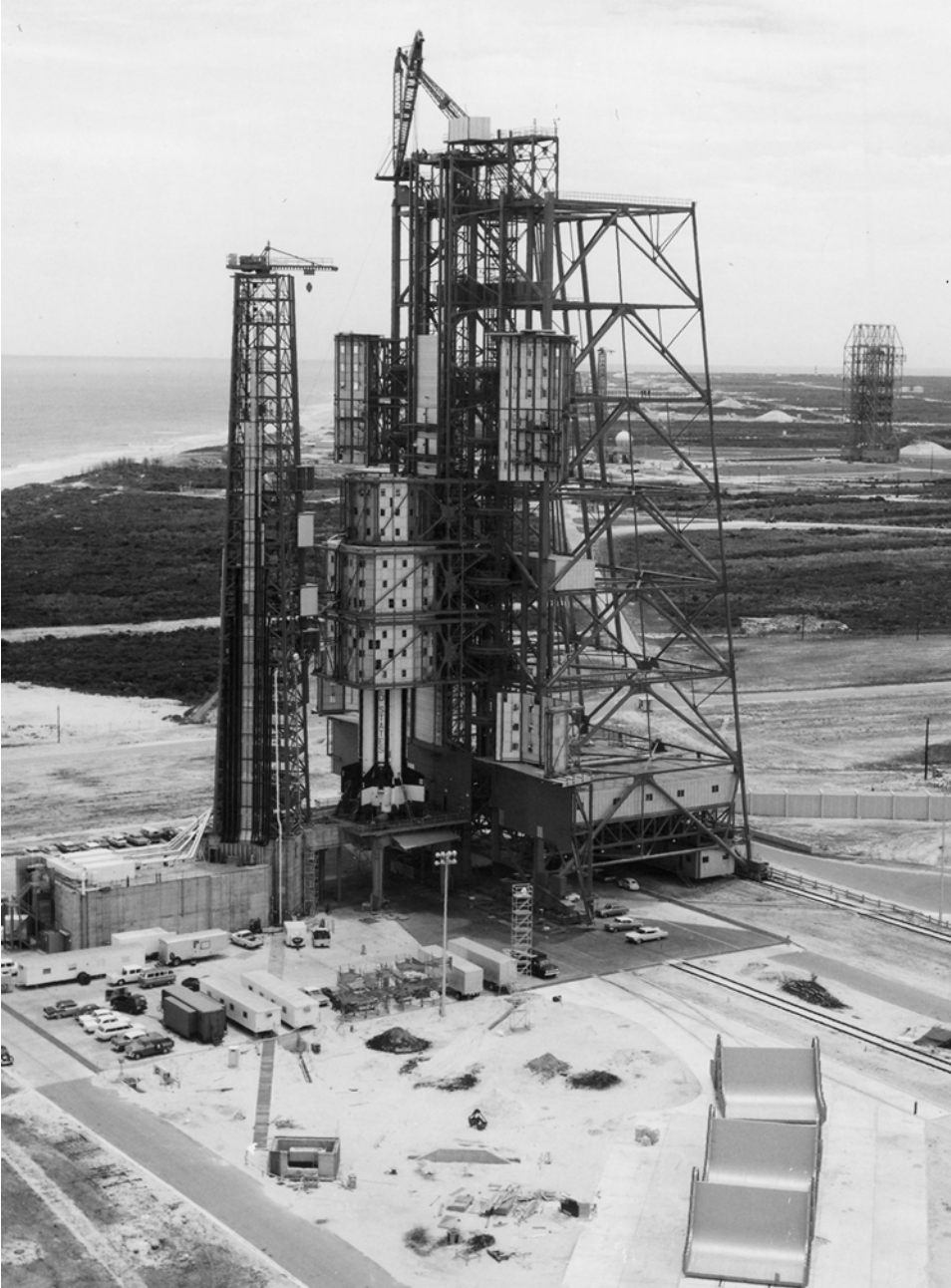
2.11 SA-5 being stacked on pad 37B. Three of the service structure's clamshells enclose the vehicle, and two are open. The LC-34 service structure is visible in the background at right. Source: NASA/Jerome Bascom-Pipp
