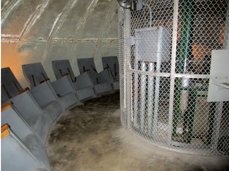
8.24 The interior of the pad A blast room. The cage in the center of the room held food and other supplies. The floor was mounted on springs to absorb shock from explosions on the pad (Photo by the author, August 2013). Source: Ward
