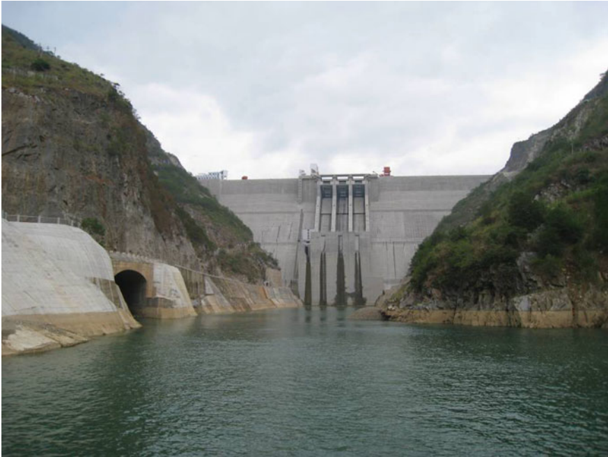
Fig. 17.35 Guangzhao Dam in service (2009-10-04)
