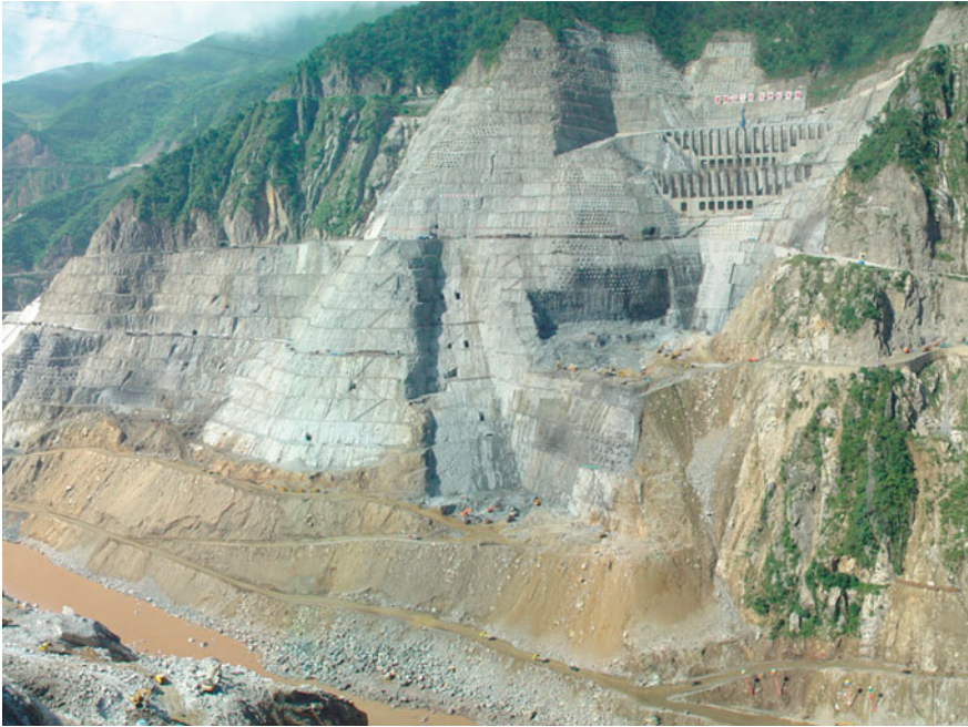
Fig. 8.13 Right abutment excavation (2004–12)
