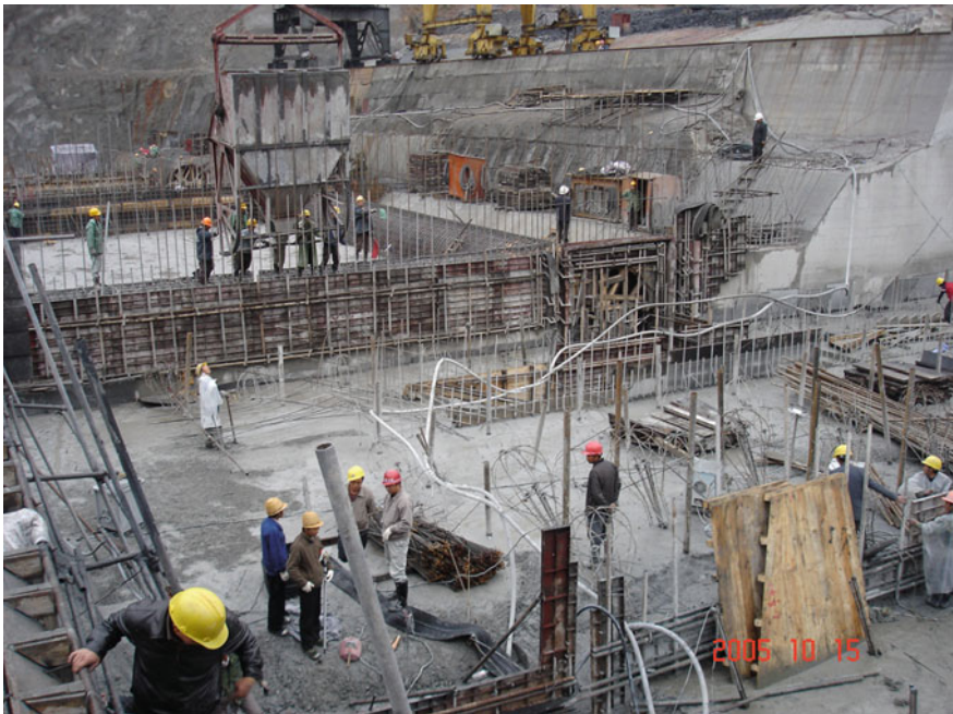
Fig. 6.45 Rock bolts under the construction
