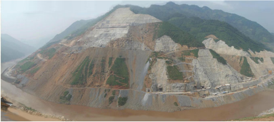
Fig. 6.31 Downstream-right bank view of the intake slope (cut elevation 440 m)
