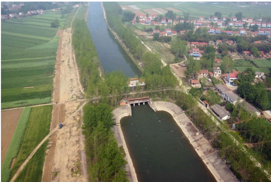
Fig. 16.25 Bird eye view of Luohansi Sluice, China
