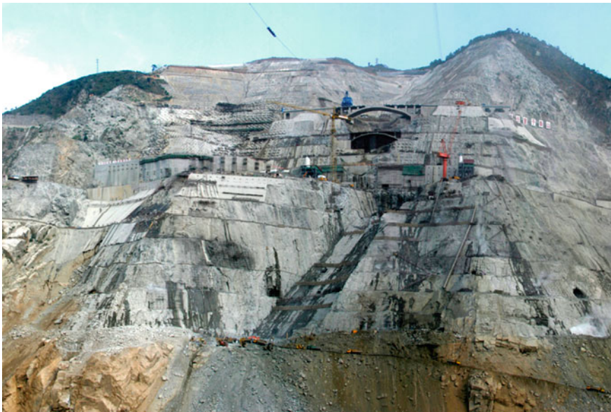
Fig. 8.12 Left abutment excavation (2004–12)
