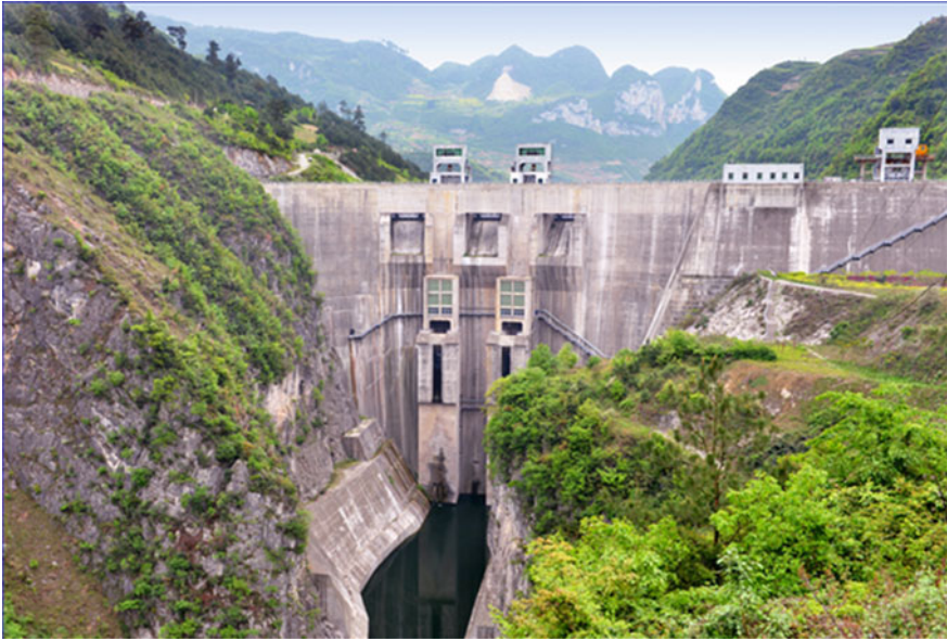
Fig. 11.21 Dahuashui Project in service (downstream view)
