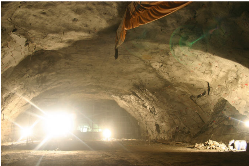
Fig. 6.27 Generator chamber after the bench I
