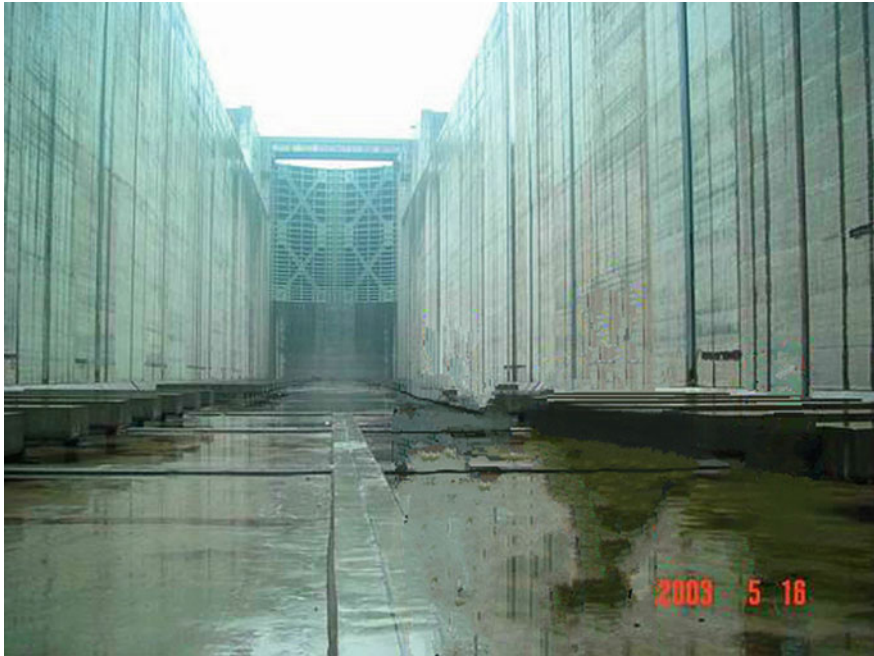
Fig. 7.27 Accomplished ship lock: Three Gorges Project, China
