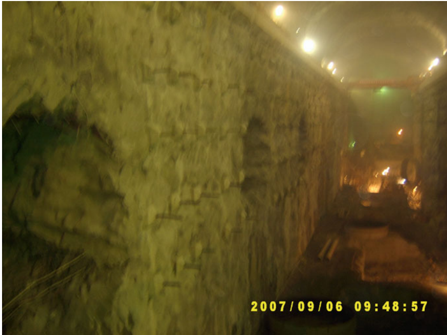
Fig. 6.28 Generator chamber after the bench VIII
