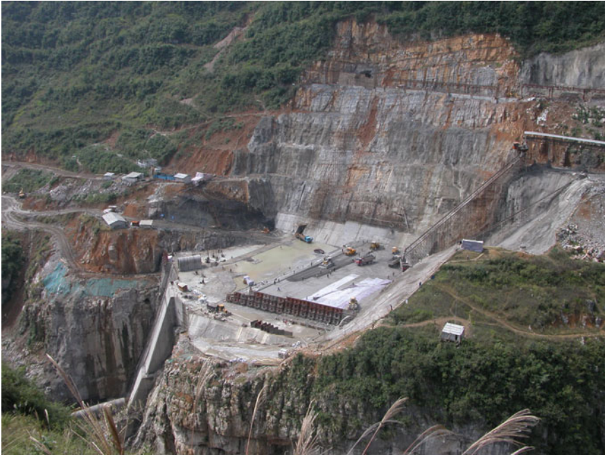
Fig. 11.9 Start of the gravity pier construction
