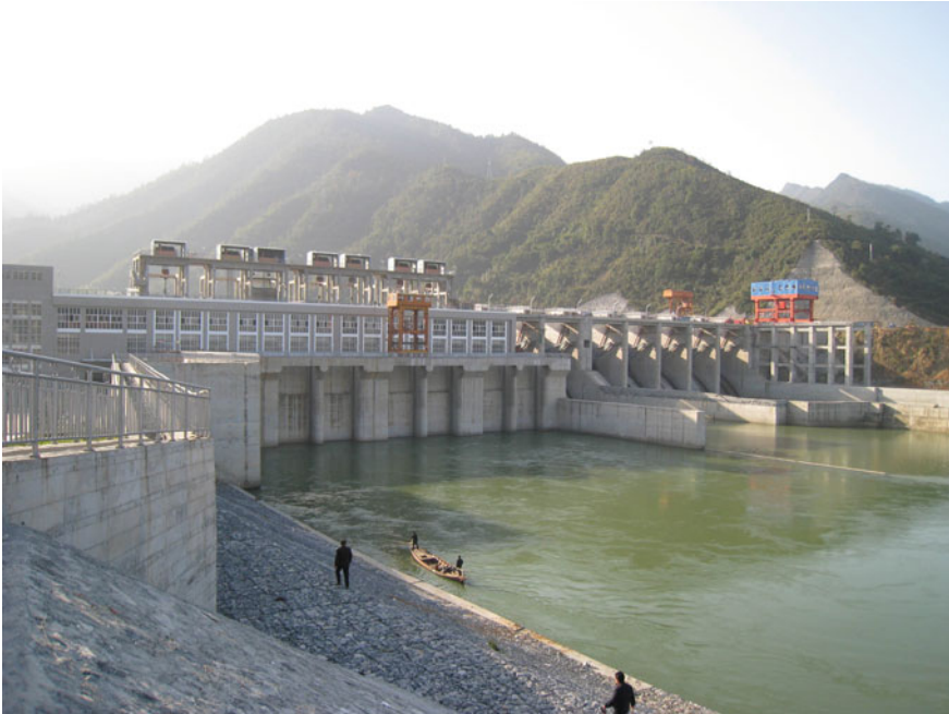
Fig. 6.48 Xiaoxi project in service
