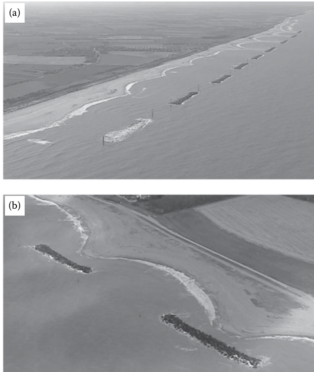
Figure 9.16 Detached Breakwater schemes at (a) Happisburgh to Winterton (stage two in foreground and stage one in distance) and (b) Elmer.
