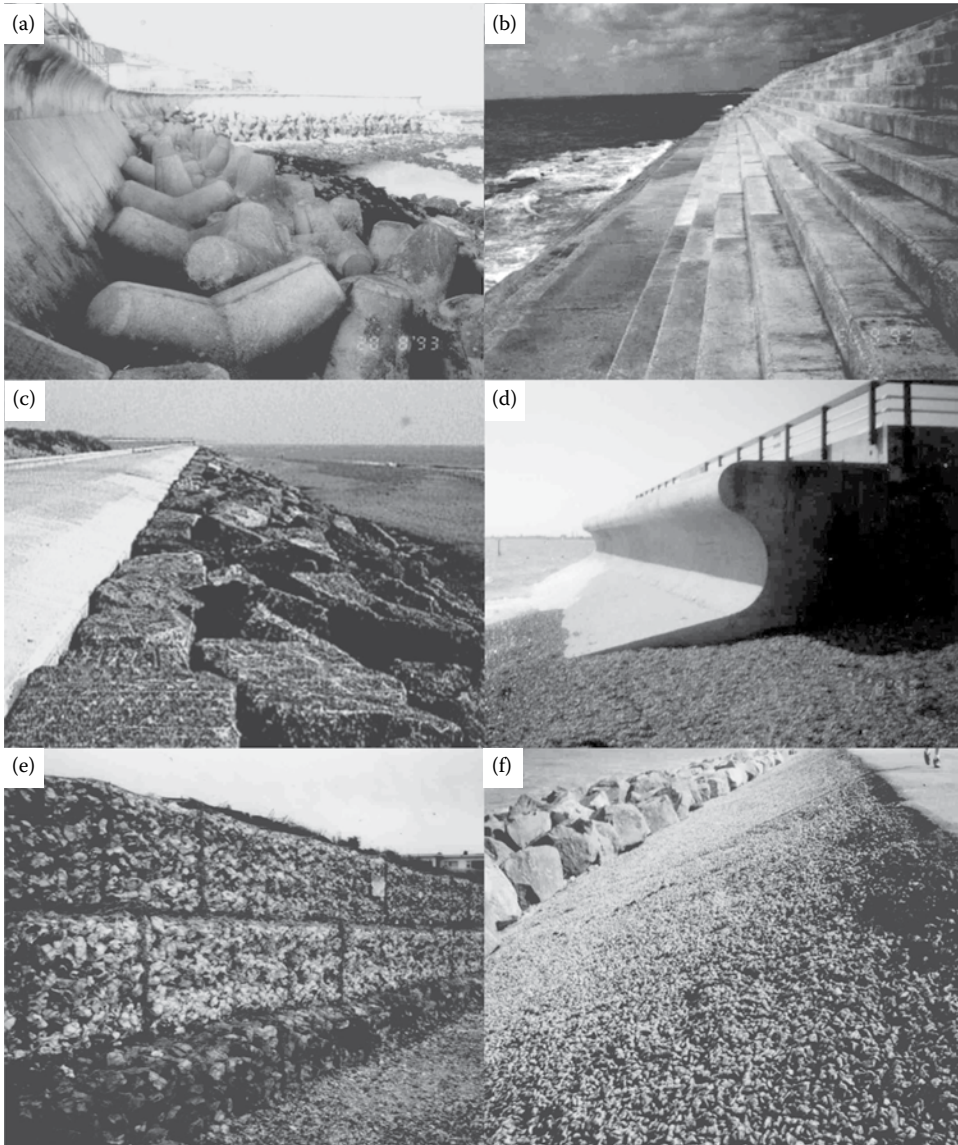
Figure 9.25 Examples of sea wall types (a) Tetrapod toe, (b) Stepped, (c) Rock toe, (d) Recurved wall, (e) Gabions and (f) Open stone asphalt with rock toe.
