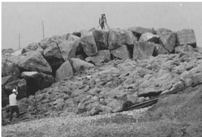
Figure 9.44 Primary armour and underlayer under construction.
