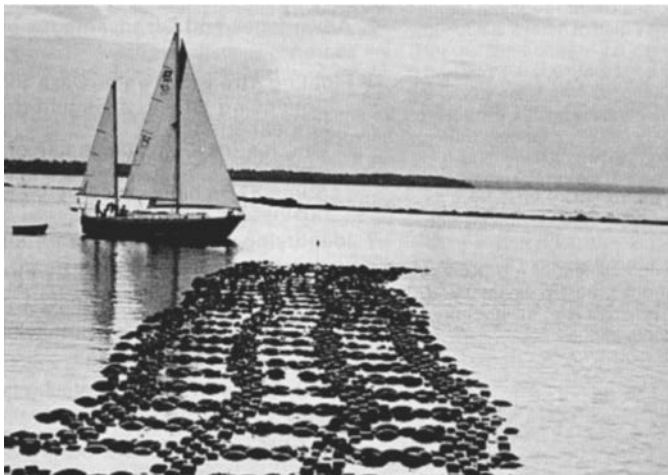
Figure 9.24 Floating tyre breakwater.
