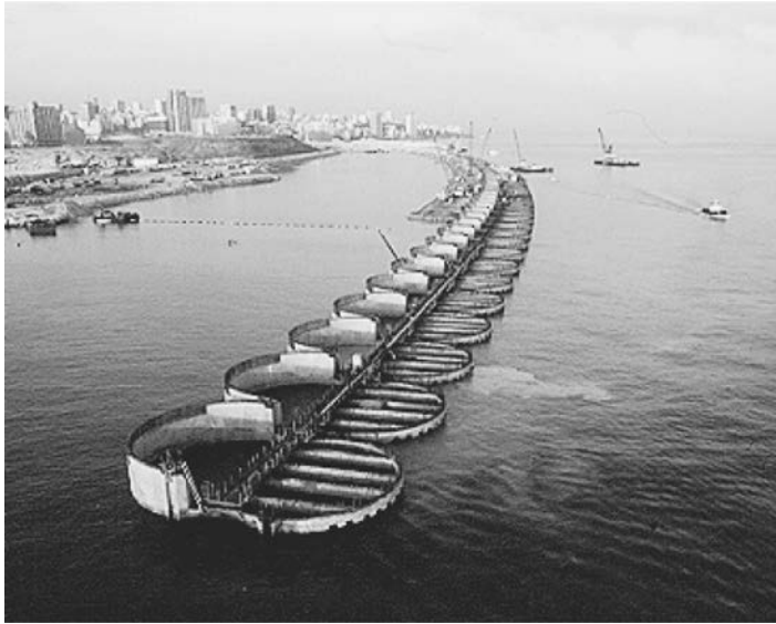
Figure 9.22 Caisson breakwater under construction.
