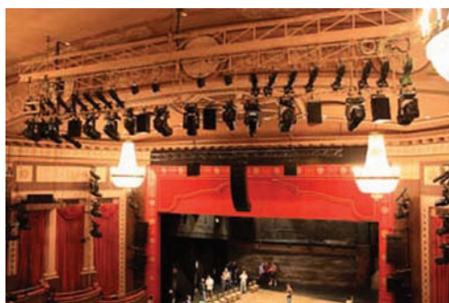
6.6.3 Circle front sound rigging: 'Billy Elliot' Imperial Theater New York, USA Photograph: John Owens
