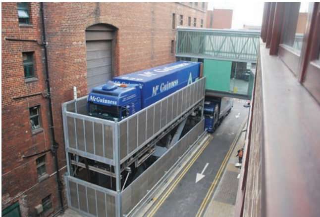
7.3.4 A vehicle lift at the Grand Theatre and Opera House, Leeds, UK Photograph: Ric Green courtesy of Opera North
