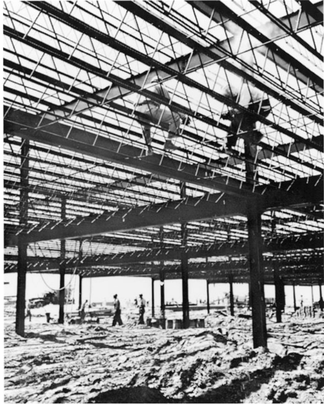
Short-span joists in the Univac Center of Sperry-Rand Corporation, Blue Bell, PA. (Courtesy of Bethlehem Steel Corporation.)
