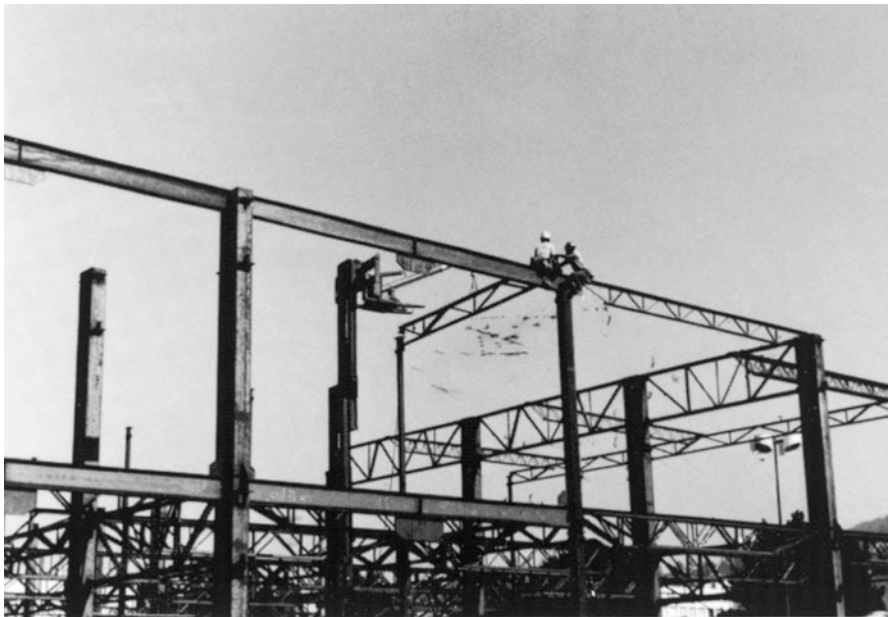
Erection of steel joists. (Courtesy of Vulcraft.)
