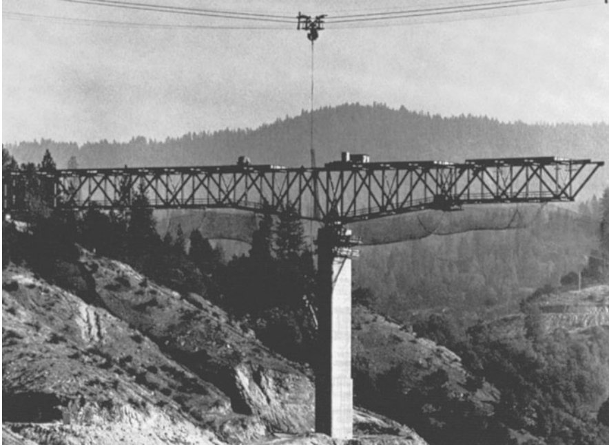
South Fork Feather River Bridge in northern California, being erected by use of a 1626-ft-long cableway strung from 210-ft-high masts anchored on each side of the canyon. (Courtesy of Bethlehem Steel Corporation.)
