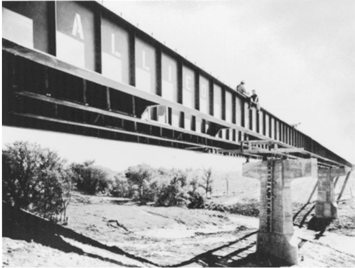
Continuous-welded plate girders in Henry Jefferson County, IA. (Courtesy of the Lincoln Electric Company.)
