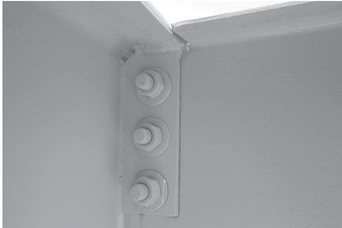
A shear tab, or single-plate, framing connection. (Picture taken by the author.)
