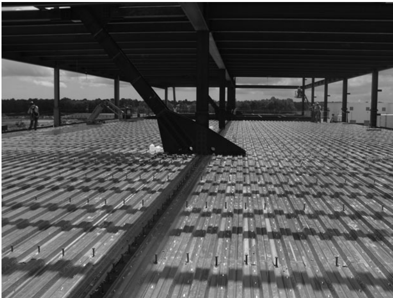
Composite floor framing, North Charleston, SC. (Courtesy of CMC South Carolina Steel.)
