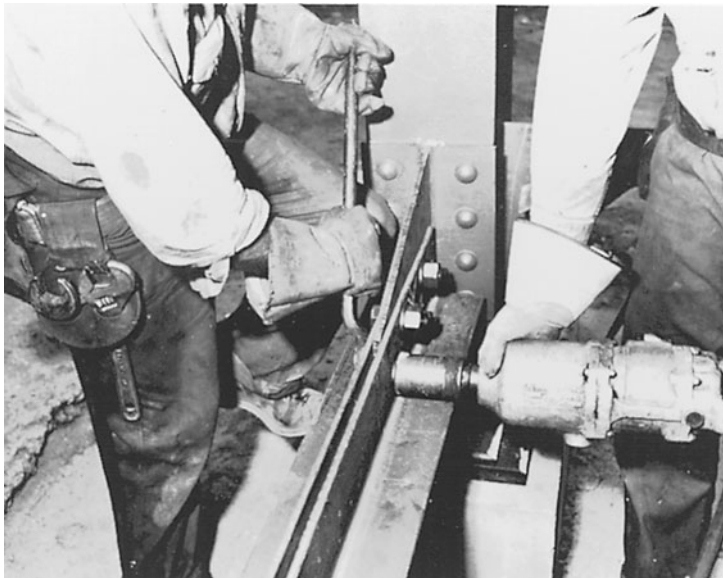
Torquing the nut for a high-strength bolt with an air-driven impact wrench. (Courtesy of Bethlehem Steel Corporation.)
