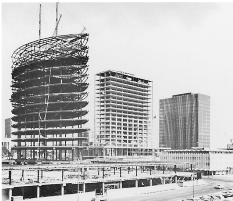
Three high-strength bolted structures in Constitution Plaza Complex, Hartford, CT, using approximately 195,000 bolts. (Courtesy of Bethlehem Steel Corporation.)
