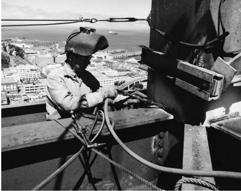
Combined welded and bolted joint, Transamerica Pyramid, San Francisco, CA. (Courtesy of Kaiser Steel Corporation.)
