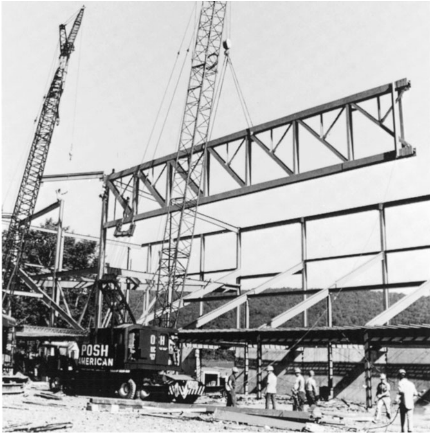
One-half of a 170-ft clear span roof truss for the Athletic and Convention Center, Lehigh University, Bethlehem, PA. (Courtesy of Bethlehem Steel Corporation.)
