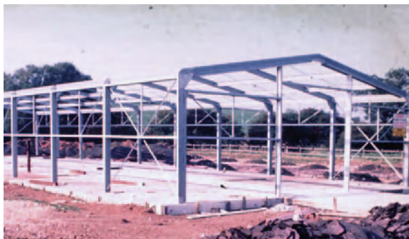
Fig. 1.2 Cold-formed steel portal framing system
