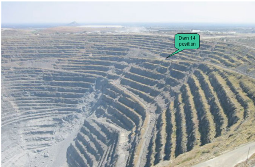
Fig. 7.57 Start of the North Wall failure—September 2004
