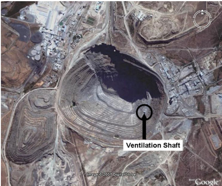
Fig. 7.56 Position of the Ventilation Shaft
