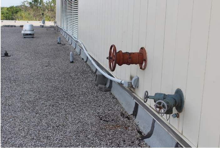
Fig. 4.18 Roof manifold
