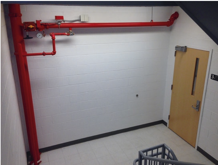
Fig. 4.8 Separate riser for sprinkler system in same stairwell as standpipe system shown in Fig. 4.7
