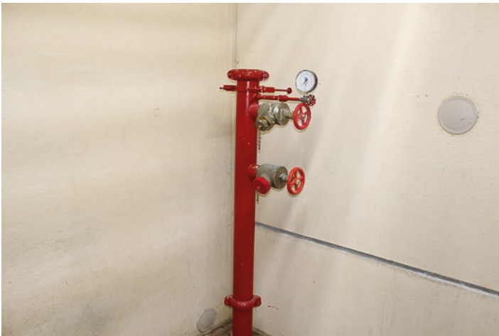
Fig. 4.19 Two outlets at a remote location to facilitate testing
