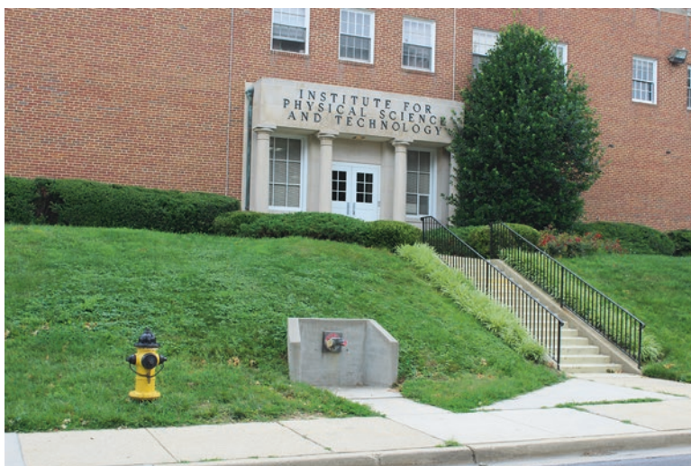
Fig. 5.20 FDC away from building near fire hydrant
