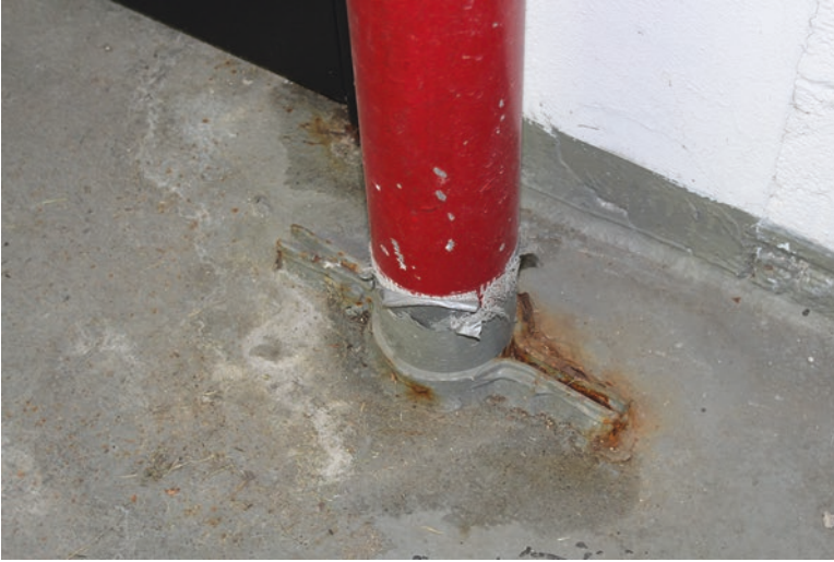
Fig. 14.4 Corrosion on a vertical standpipe support
