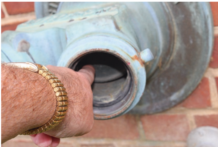
Fig. 14.3 Checking the clapper in an FDC
