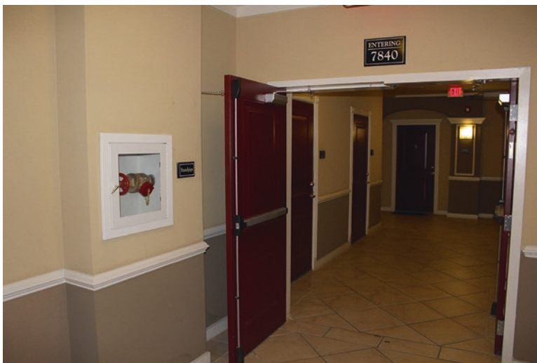
Fig. 4.11 Horizontal exit and Class I standpipe hose connection
