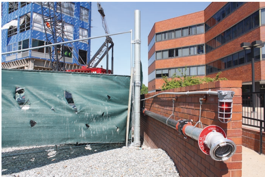
Fig. 1.6 Fire department connection for standpipe system in building under construction. Note: Photo taken by Paul Drougas, used with permission
