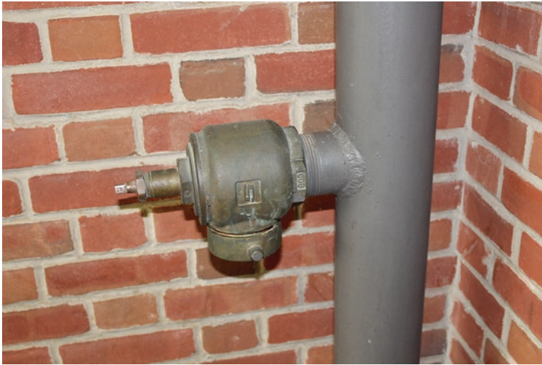
Fig. 14.1 Standpipe hose connection valve missing a valve handle
