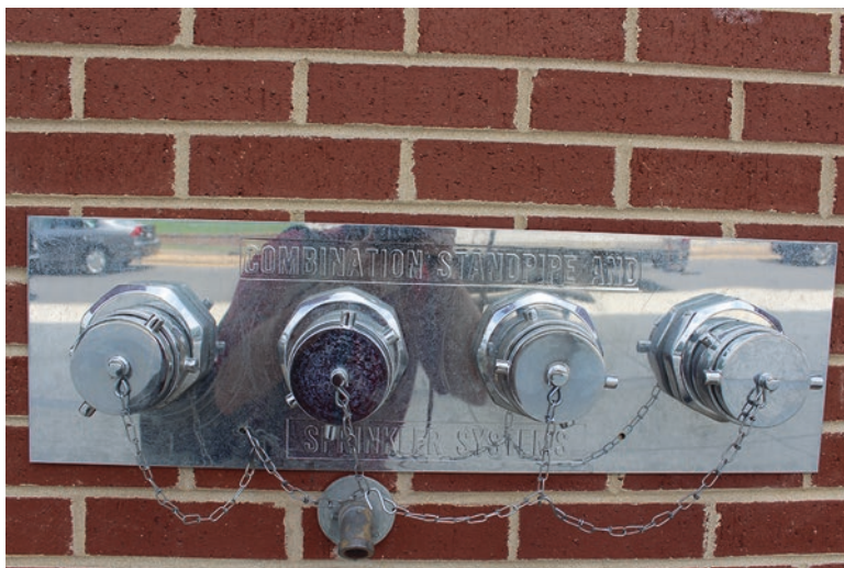
Fig. 5.15 A fire department connection for a standpipe system with a demand of 1000 gpm and four inlet connections
