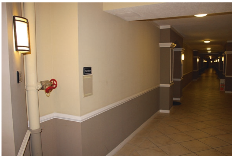
Fig. 4.21 Class I outlet in hallway because outlets in stairs were too far from remote points in building
