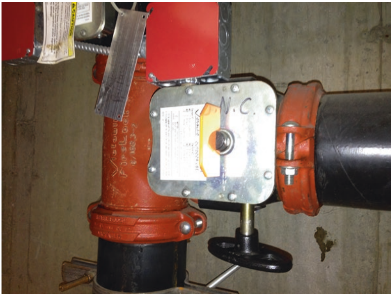
Fig. 5.8 Butterfly valve with paddle perpendicular to pipe indicating water cannot flow
