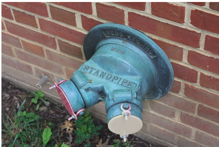
Fig. 5.14 A fire department connection with two 2.5 in. inlet connections
