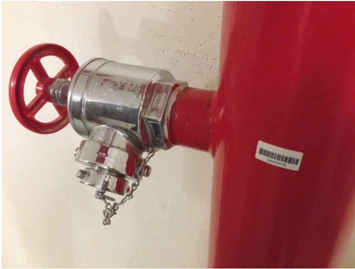
Fig. 14.10 Bar code used to keep track of inspection, testing and maintenance of a hose connection on a Class III standpipe system
