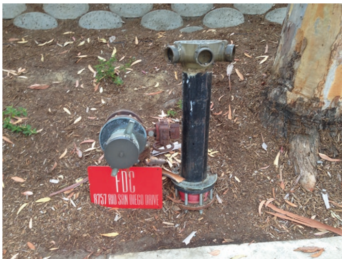
Fig. 5.16 Large diameter threadless coupling used as fire department connection for a standpipe system
