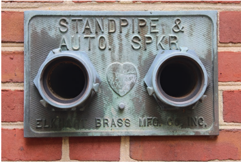
Fig. 14.2 Missing cap on standpipe FDC
