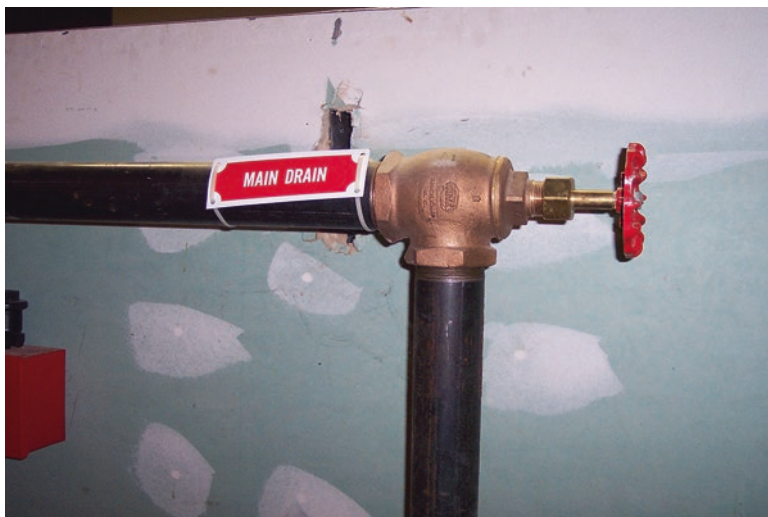
Fig. 14.5 Two-inch main drain connection
