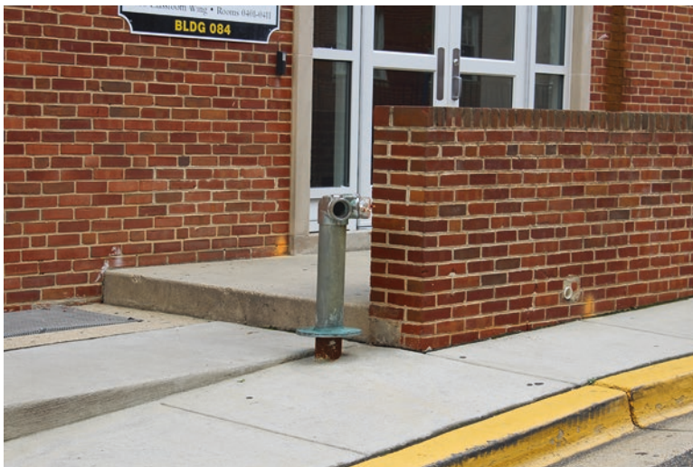
Fig. 5.21 FDC on a freestanding post away from the building to keep egress clear
