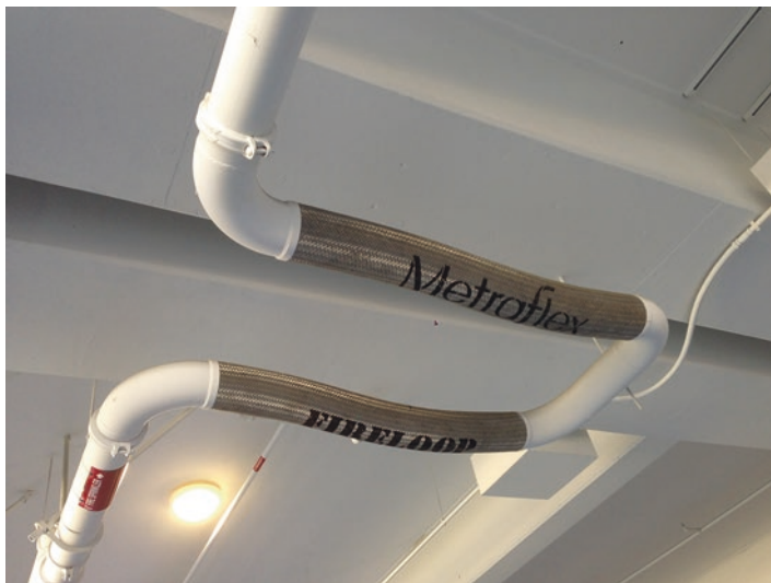
Fig. 11.12 Seismic separation assembly for standpipe system
