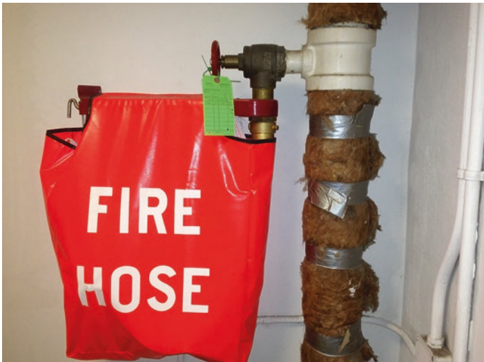
Fig. 2.8 Class II standpipe system
