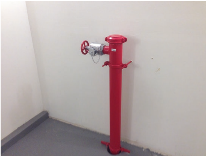
Fig. 2.11 Class III standpipe without hose
