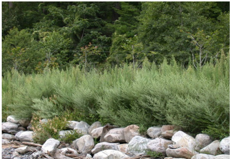
Fig. 4 Constructed bank formed of natural abiotic and live material
