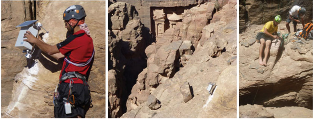
Fig. 15 Installation of wireless instrumentation network (Delmonaco et al. 2014)
