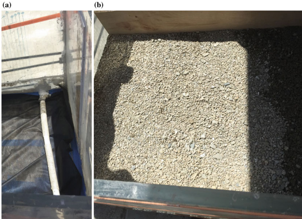
Fig. 1 a Perforated pipe installed at the base of the Plexiglass container and b gravel layer compacted above the perforated pipe to serve as a drainage layer during the model test
