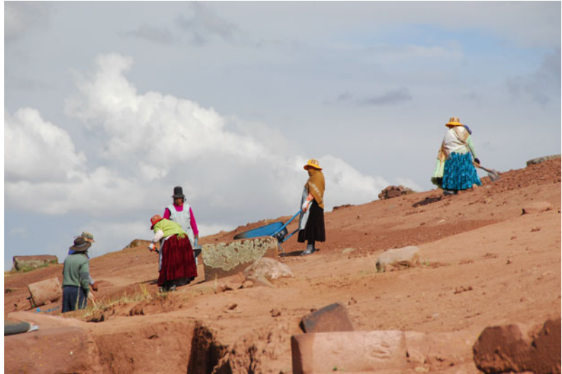
Fig. 8 Protecting a pyramid earth mound from soil erosion by means of penka
