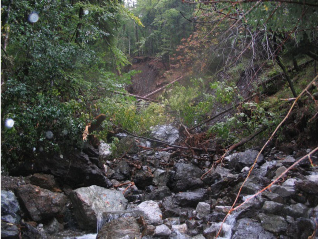
Fig. 8 Debris flow deposition in the watershed of the Hrenovec torrent
