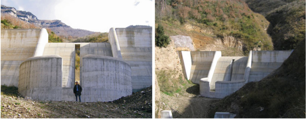
Fig. 9 Upstream open check dam in the Cantariello gully in Sarno
