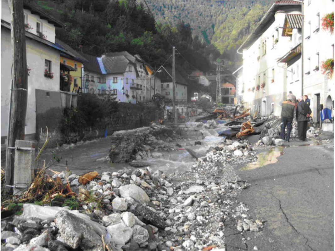
Fig. 7 Consequences of September 2007 flash flood in the centre of the Kropa village
