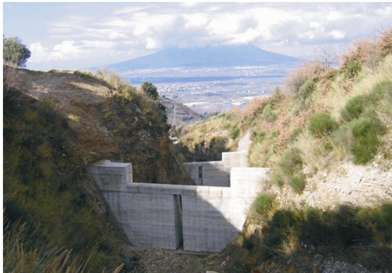
Fig. 10 Check dams in the Cantariello gully in Sarno
