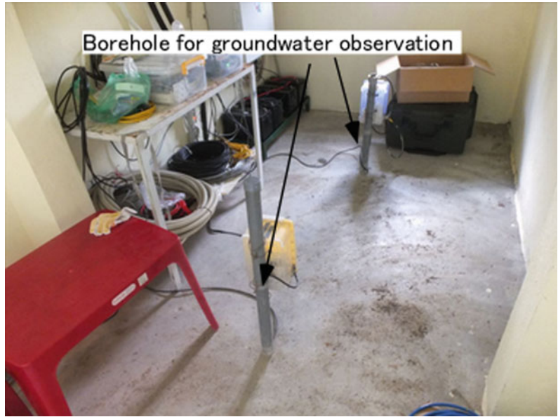
Fig. 6 Groundwater pressure gauge setting condition
