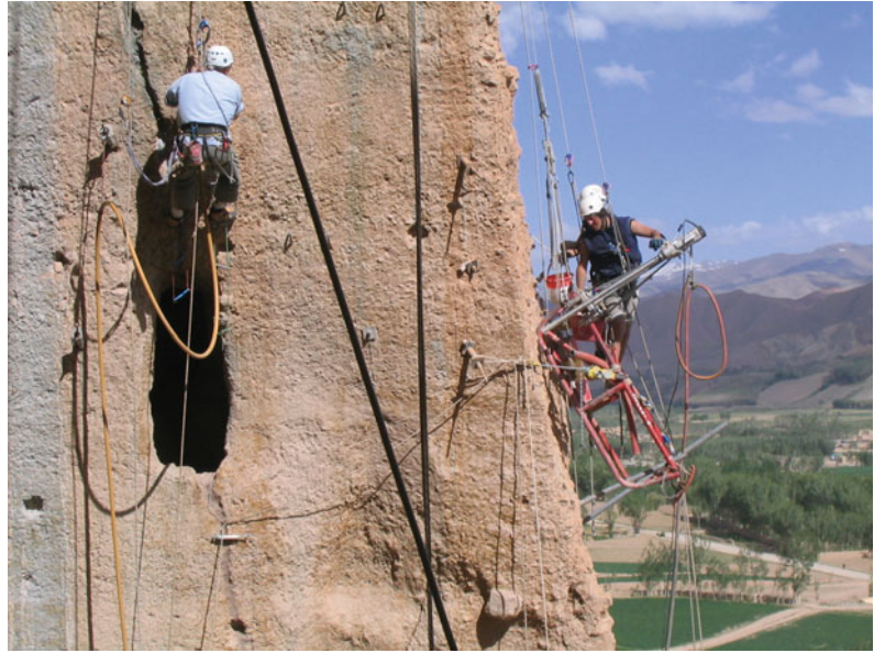
Fig. 9 Execution of anchors and nails for the stabilisation of unstable blocks
