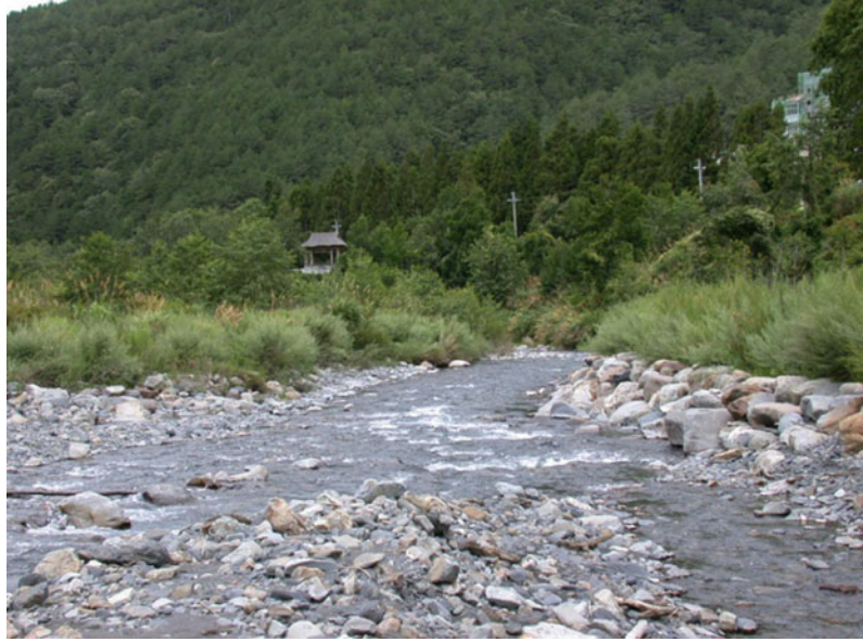
Fig. 5 Constructed stream bank ( right ) versus a natural bank ( left )
