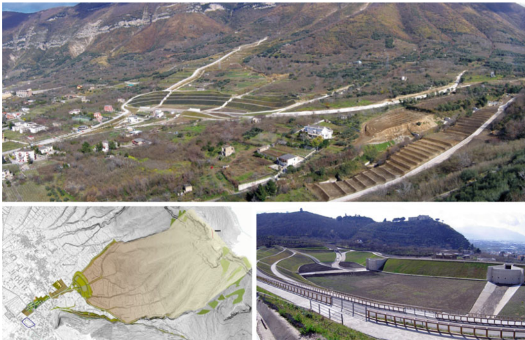
Fig. 5 In the upper picture a large view of the single basin system, in Episcopio (Sarno). Down-left the drawing shows the area of potential flows from the slopes which converge in the tank; down-right a photographic detail inside the tank
