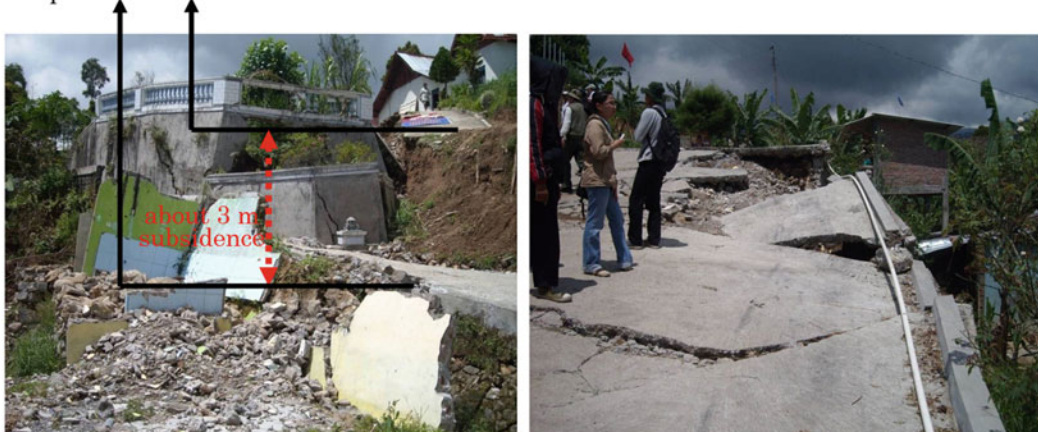
Fig. 1 The impacts of landslide Tengklik Village, landsubside and the damage of houses and main road (Karnawati et al. 2009a)
