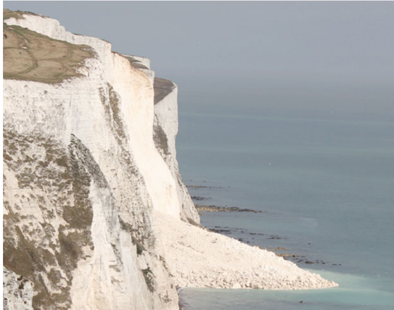
Fig. 1 Chalk cliff collapse at Fan Bay, March 9th, 2012
